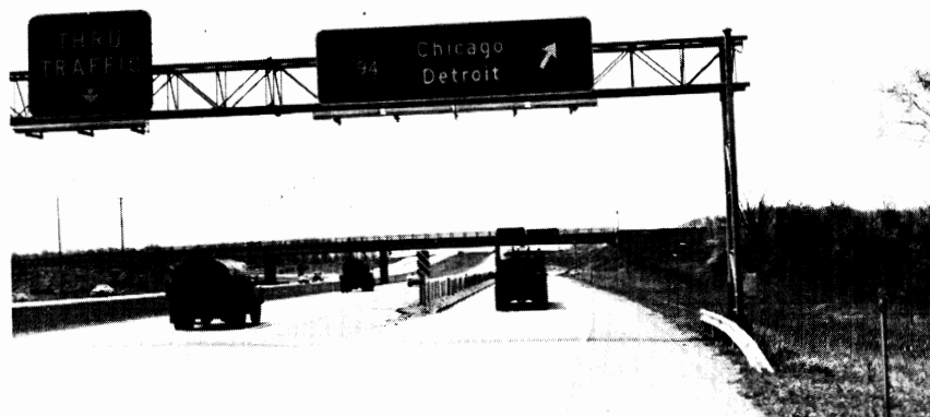
Sign 3. "Chicago," Illuminated sign, Background - 4.9 ft-L, Legend - 33 ft-L, 6.7:1, 16" - 12", V = 21.5 .
