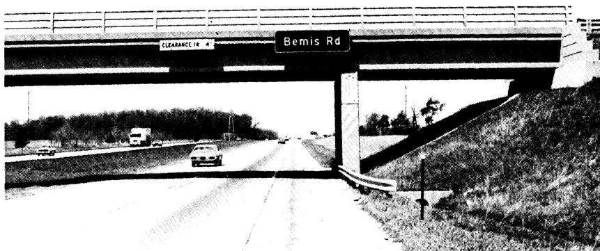
Sign 9. "Bemis Rd.," Background - 10.8 \text{ cp/ft-c/ft}^2 , Legend - 68.0 \text{ cp/ft-c/ft}^2 , 6.3:1, 13.3" - 10," V = 18.5, H = 5.
