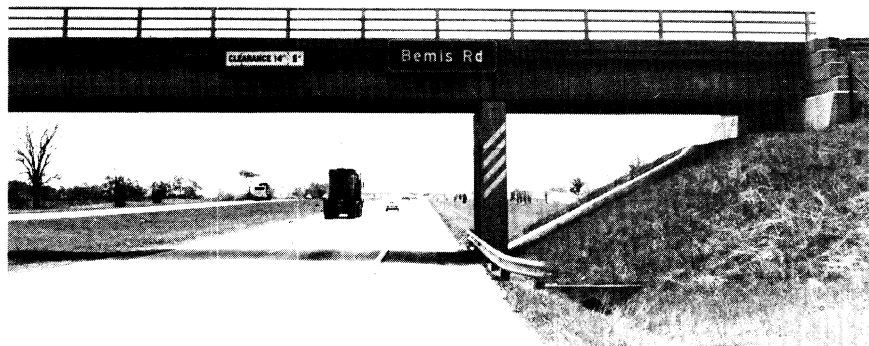
Sign 19. "Bemis Rd." Background - 0.8 \text{ cp/ft-c/ft}^2 , Legend - 12.2 \text{ cp/ft-c/ft}^2 , 14.7:1 , 13.3'' - 10'' , V = 17.5 , H = 4 .
