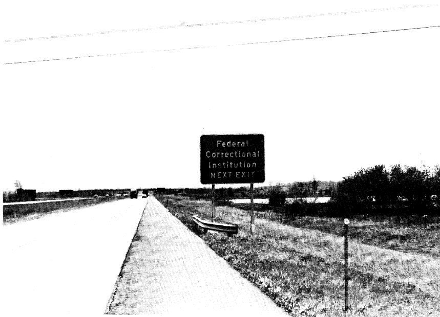
Sign 12. "Federal Correctional Institution," Background - 24.7 cp/ft-c/ft 2 , Legend - 58.7 cp/ft-c/ft 2 , 2.4:1, 13.3" - 10", V = 13.5, H = 19.
