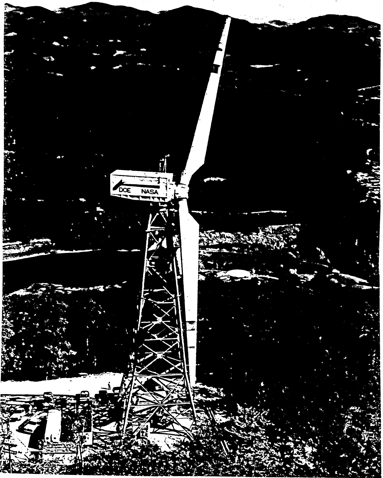
Fig. 2-3: View of the MOD-1 WT looking NE.
