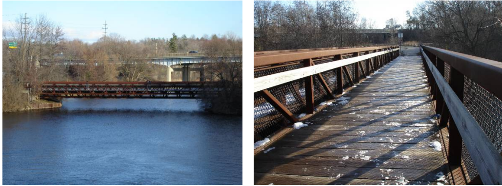
Figure 2.12: Bandemer Park pedestrian bridge.
