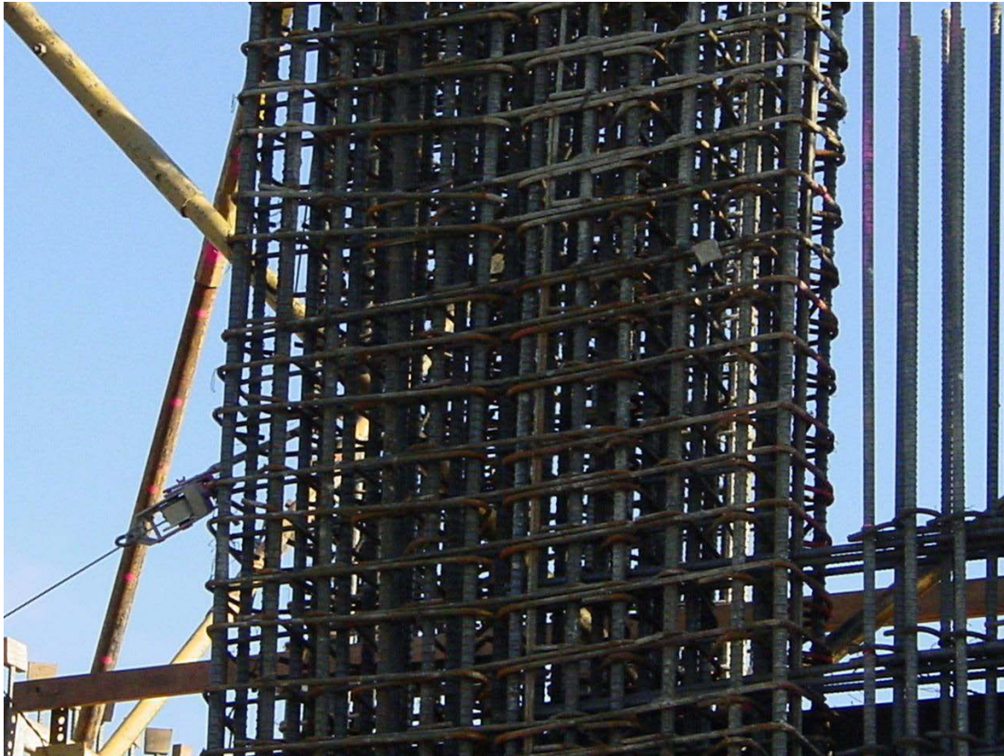
Fig. 1-1 Typical Reinforcement Detailing in the Boundary Regions of Reinforced Concrete Structural Walls (courtesy of Andres Lepage)
