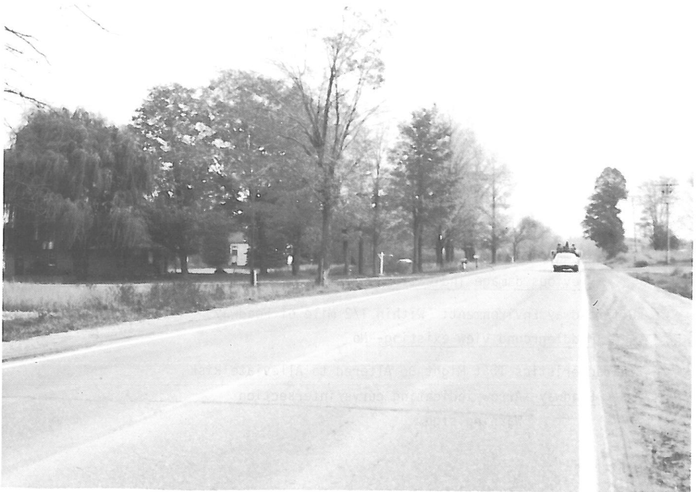
Figure A4 Scene showing typical Generic Roadside Environment 4- Trunkline/straight/urban & built-up
