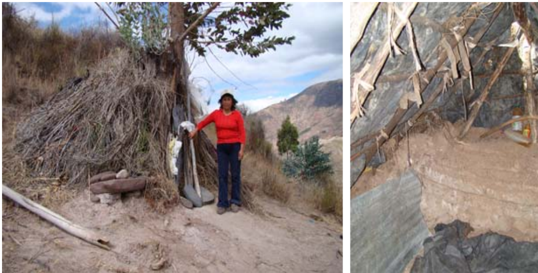
Figure 4.10: (a) Exterior and (b) interior views of a modern semi-subterranean thatched structure excavated into a hillside. Note that the simple roof was built directly on the ground surface.
