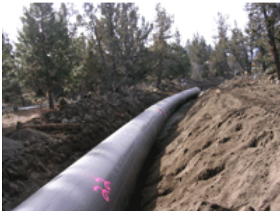
Photo 14.2: Swalley Main Canal Piping Project, Courtesy of DRC.
