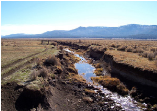
Photo 19.3: Pre-Project in 2004, Courtesy of FRCRM.
