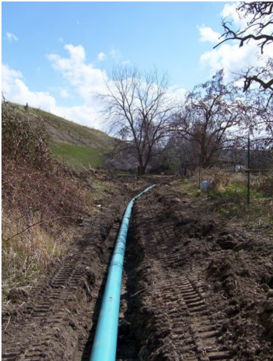
Photo 4.1: Ditch lining to reduce seepage and conserve water, Courtesy of WWWMP.
