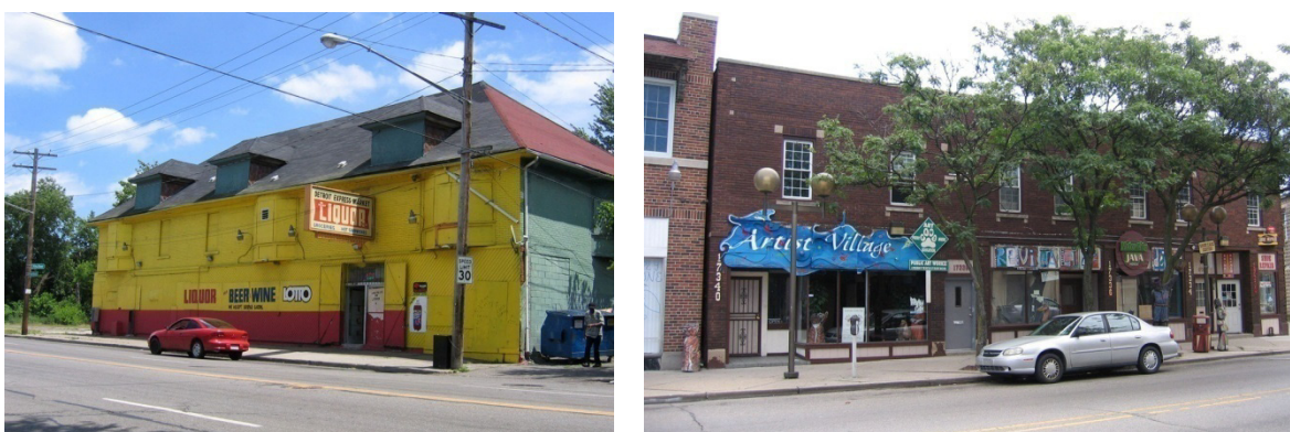
Figure 8-8 Stand-alone business establishment in a neighborhood (left) and shops in a clustering of destinations (right)
