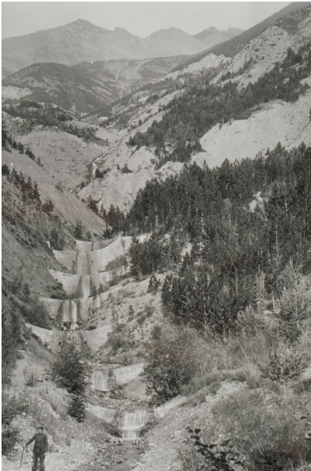
Figure 8. Restoration works on Bourget torrent
