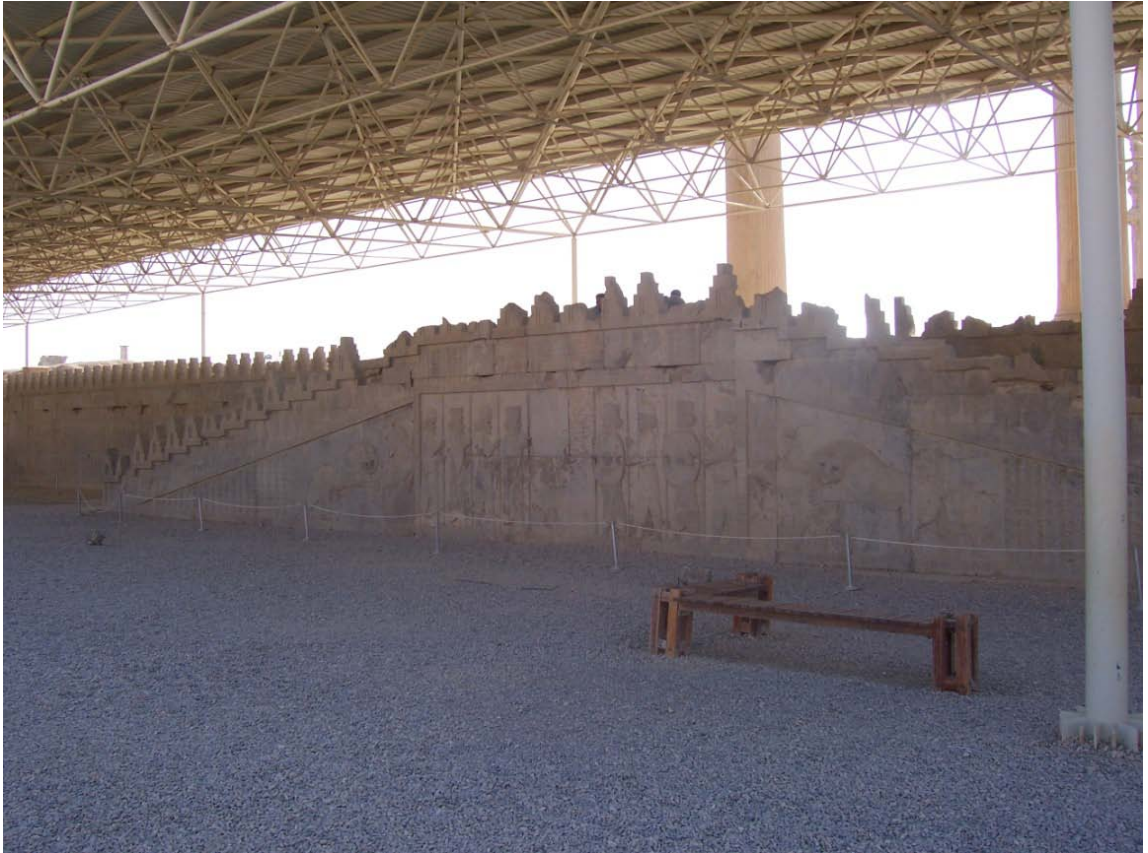
Figure 5.4 Roof above Eastern Facade of Apadana, 2009 (Photo: A. Nagel).
