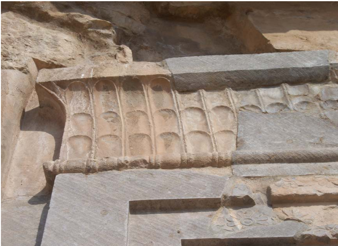
Figure 4.33 Detail of Cavetto. Façade of the Tomb of Artaxerxes II, Persepolis 2008 (Photo: A. Nagel)
