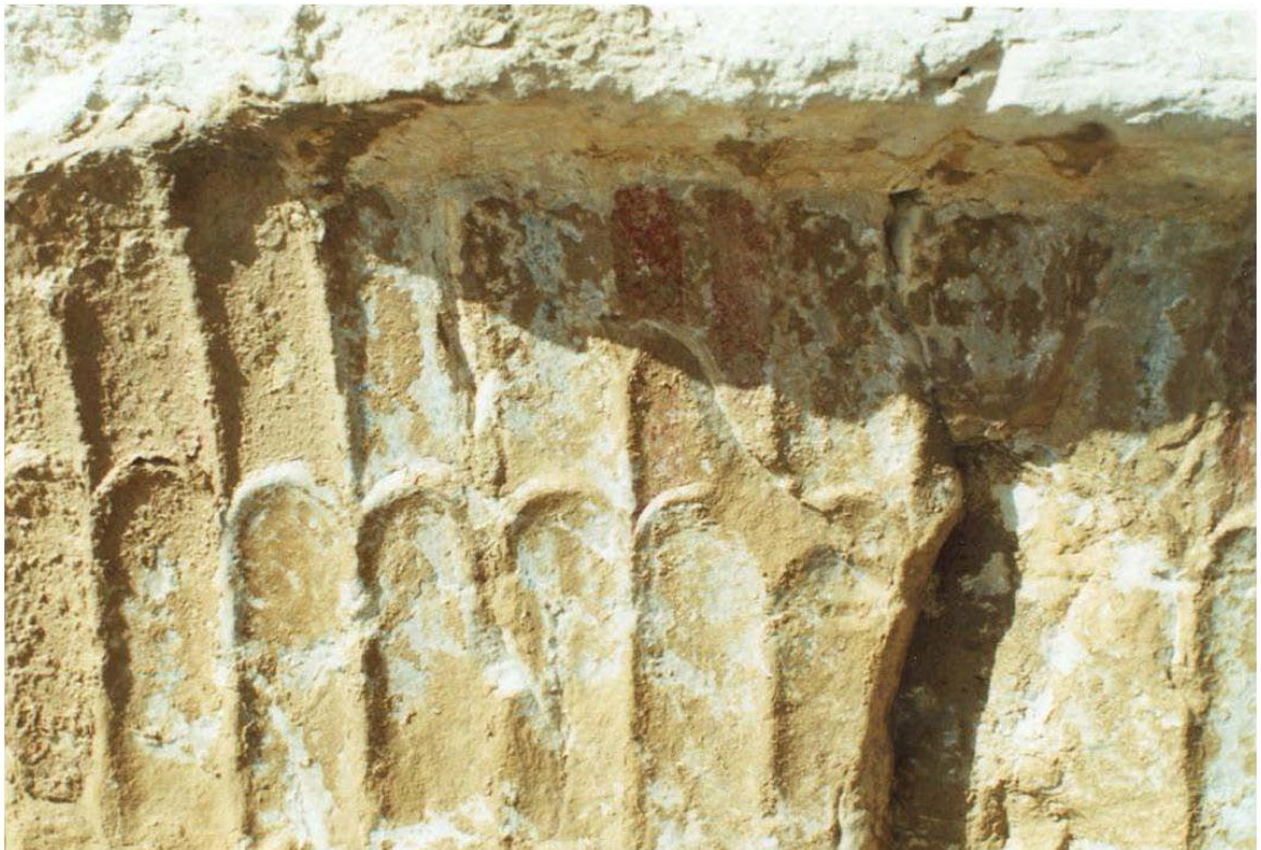
Figure 4.31 Detail of Cavetto. Façade of the Tomb of Darius I at Naqsh-e Rostam (Photo: H. Rahsaz)
