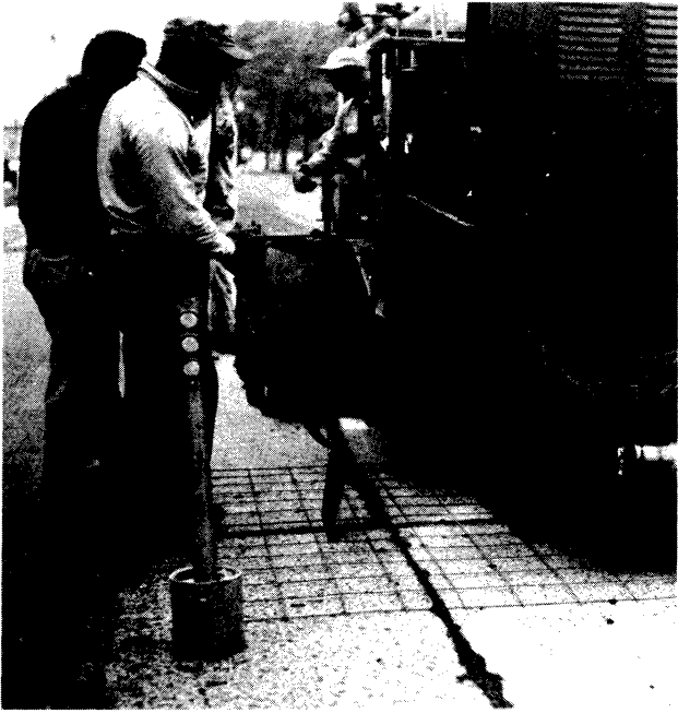
Figure 9. Typical installation of transverse reinforcing over joint.
