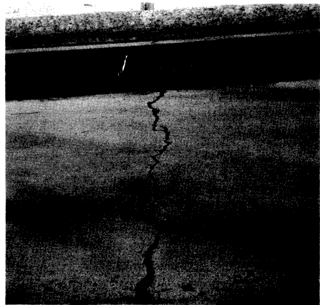
Figure 15 One of the cracks in non-reinforced section.
