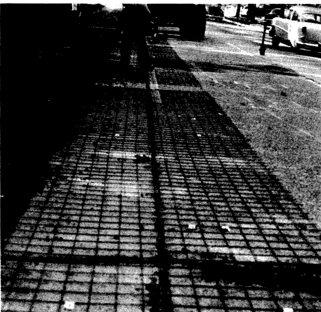
Figure 11. Typical installation of longitudinal reinforcing over joint.
