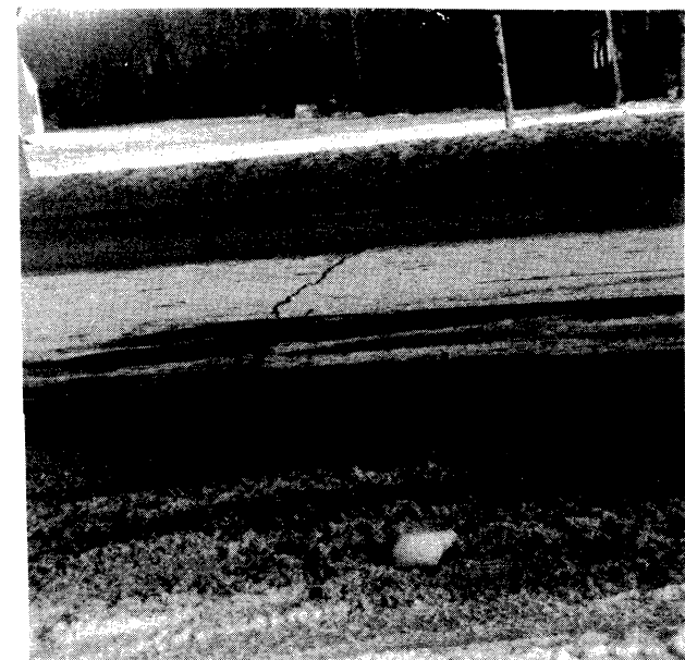
Figure 17 Crack at edge of reinforcement, Raynham.
