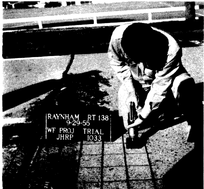
Figure 10. Remington stud driver used to hold down fabric sheets.
