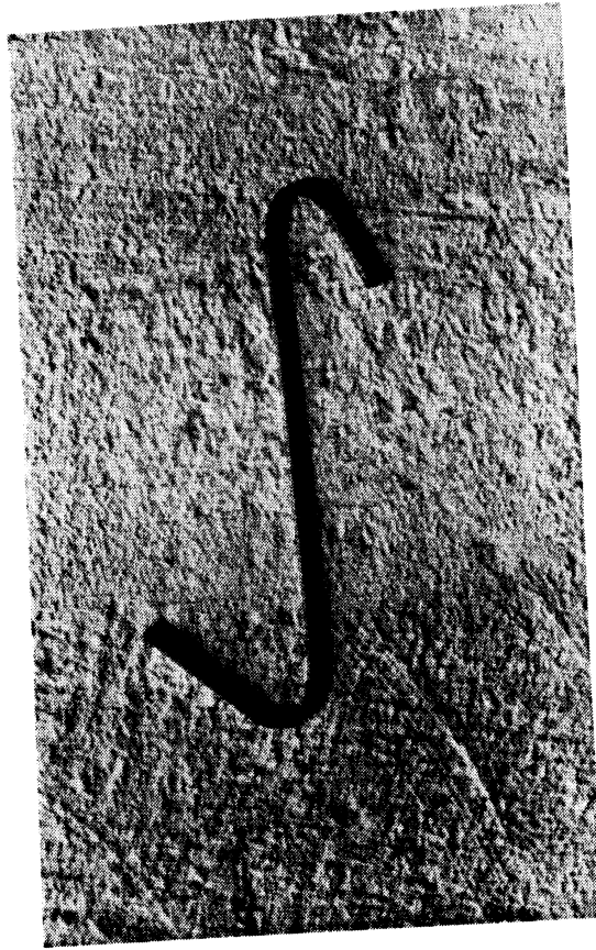
Fig. 4.9. Typical Column Cross-Tie.
