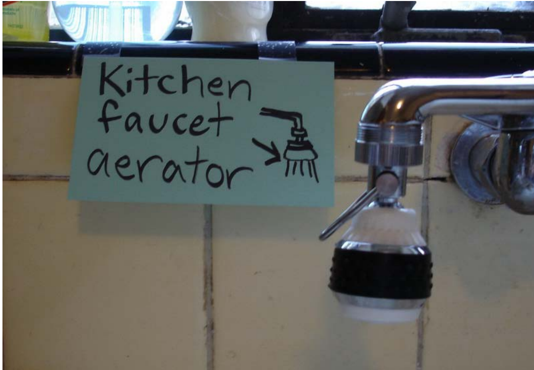
Figure 22. Signage near the kitchen sink in the Demonstration House pointing out the faucet aerator.
