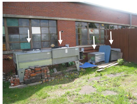
Figure 19. Outside North wall, just East of the beer garden. From left to right are the twin glycol chiller condenser fans and the two cold room chiller units
