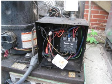
Figure 15. A motor ON/OFF state datalogger monitored the activity of the cold room chillers.
