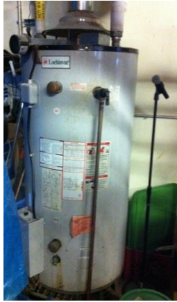
Figure 45. 200,000 BTUH domestic hot water heater
