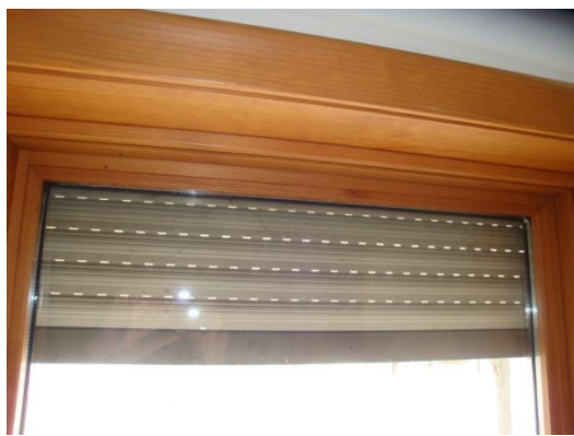
Figure 53. Inside view of shutter system. The small gaps that are visible are closed when the shade is pulled down tight, blocking all sunlight.
