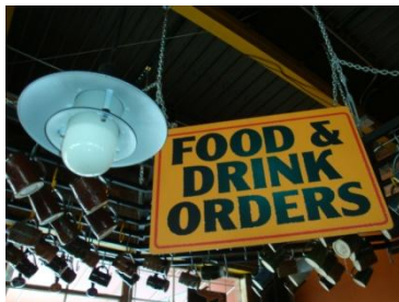
Figure 30. Lighting over bar
