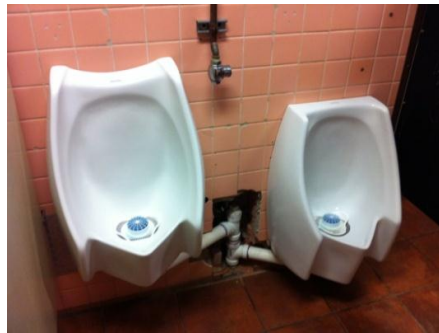
Figure 43 Waterless urinals in men's room
