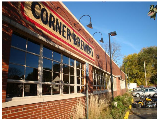
Figure 1. View of south wall
