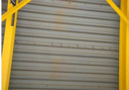
Figure 31. View of ceiling, looking upward from restaurant floor
