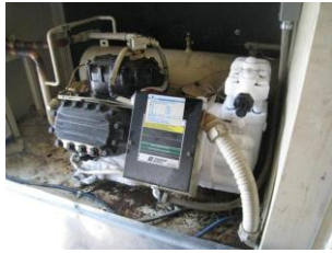
Figure 20. Glycol chiller compressor
