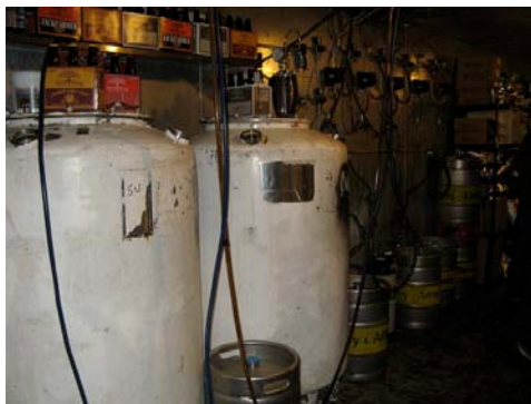
Figure 18. Walk-in cooler showing serving tanks and keg storage.
