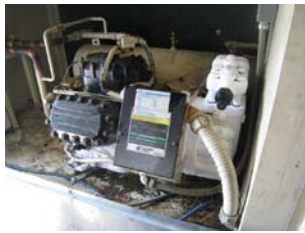
Figure 20. Glycol chiller compressor
