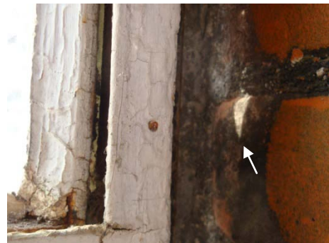
Figure 52. South-facing window detail shows sunlight passing through gap between sash and frame
