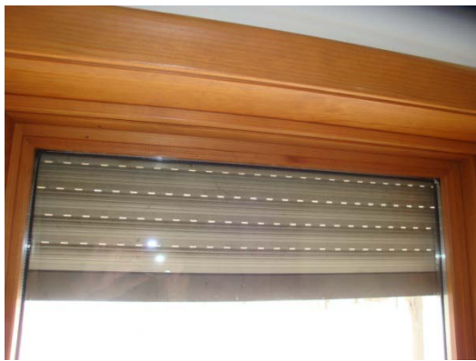
Figure 53. Inside view of shutter system. The small gaps that are visible are closed when the shade is pulled down tight, blocking all sunlight.
