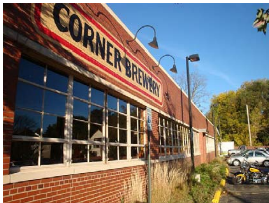
Figure 1. View of south wall
