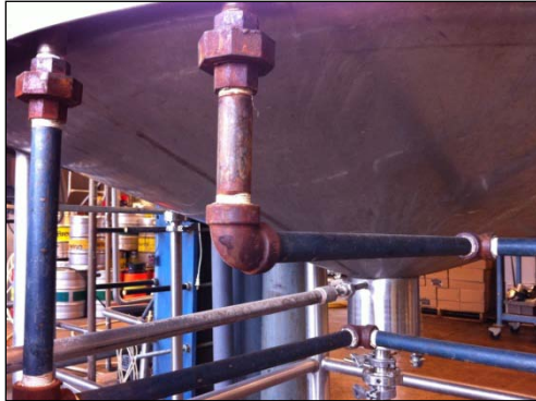
Figure 48. Uninsulated steam pipes are a big energy loser
