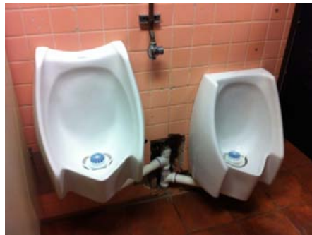
Figure 43 Waterless urinals in men's room
