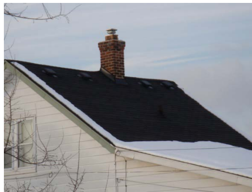
Figure 33. The snow has melted off this poorly insulated neighbor's roof, but remains on the overhanging eaves
