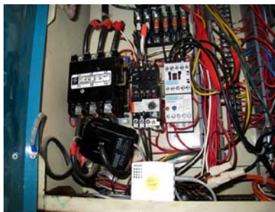
Figure 16. Chiller compressor current was measured over a several month period using a datalogger and current amplifier clamp.
