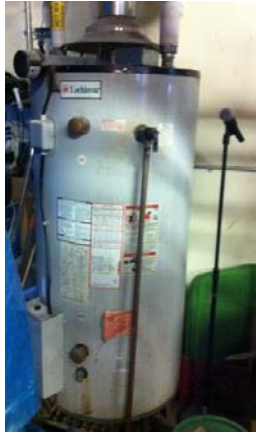
Figure 45. 200,000 BTUH domestic hot water heater
