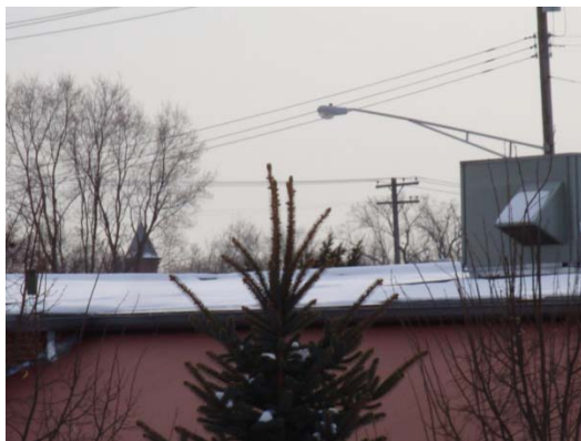
Figure 32. Accumulated snow on the roof of the Corner Brewery
