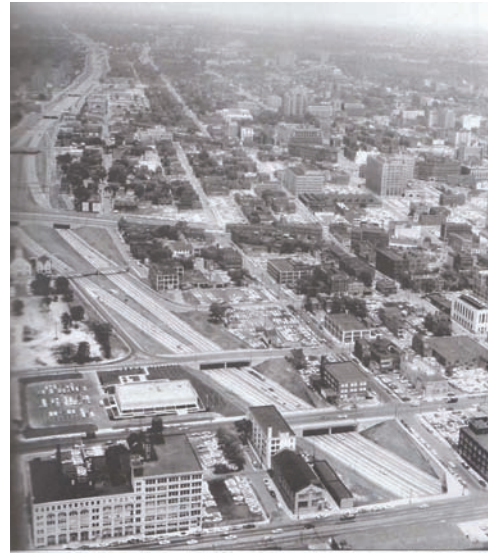
2.27 Urban renewal projects like the construction of the Lodge Freeway destroyed neighborhoods
