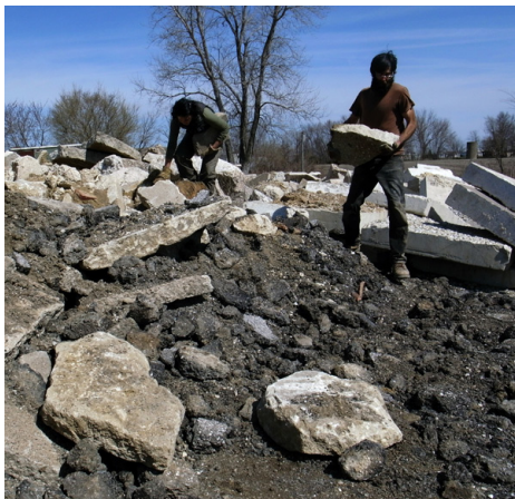
3.29 Recycling concrete for planter beds
