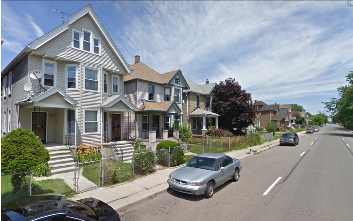
1.34 Stable block condition in study area
