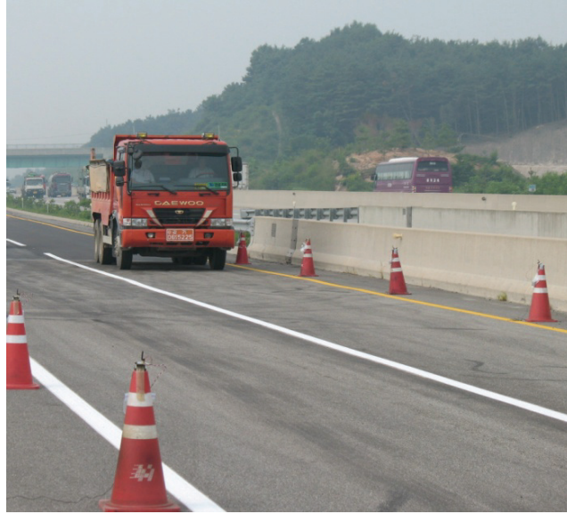
Figure 2.8 Vibrations introduced into the Yeondae Bridge using a heavy 3-axle truck driving at constant speeds over the bridge.
