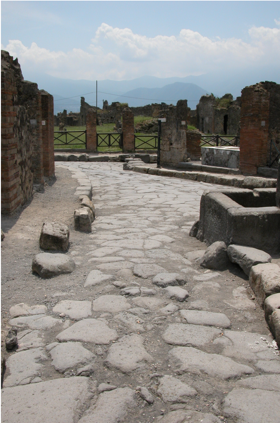
a: View south into house VII.6.7 through the main entry, from the perspective of a person standing on Vico di Modesto , just north of the fountain at the south end of insula VI.3 (to the right). The house suffered heavy damage from bombing in World War II. The niche shrine and almost the entire peristyle were destroyed.
