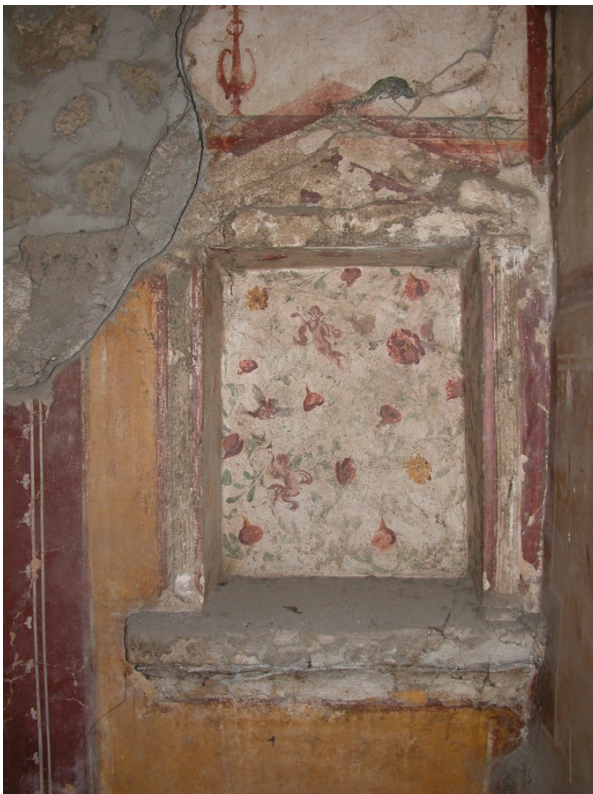
b: Painted niche with aedicula façade in the room north of the tablinum in house II.9.4.
