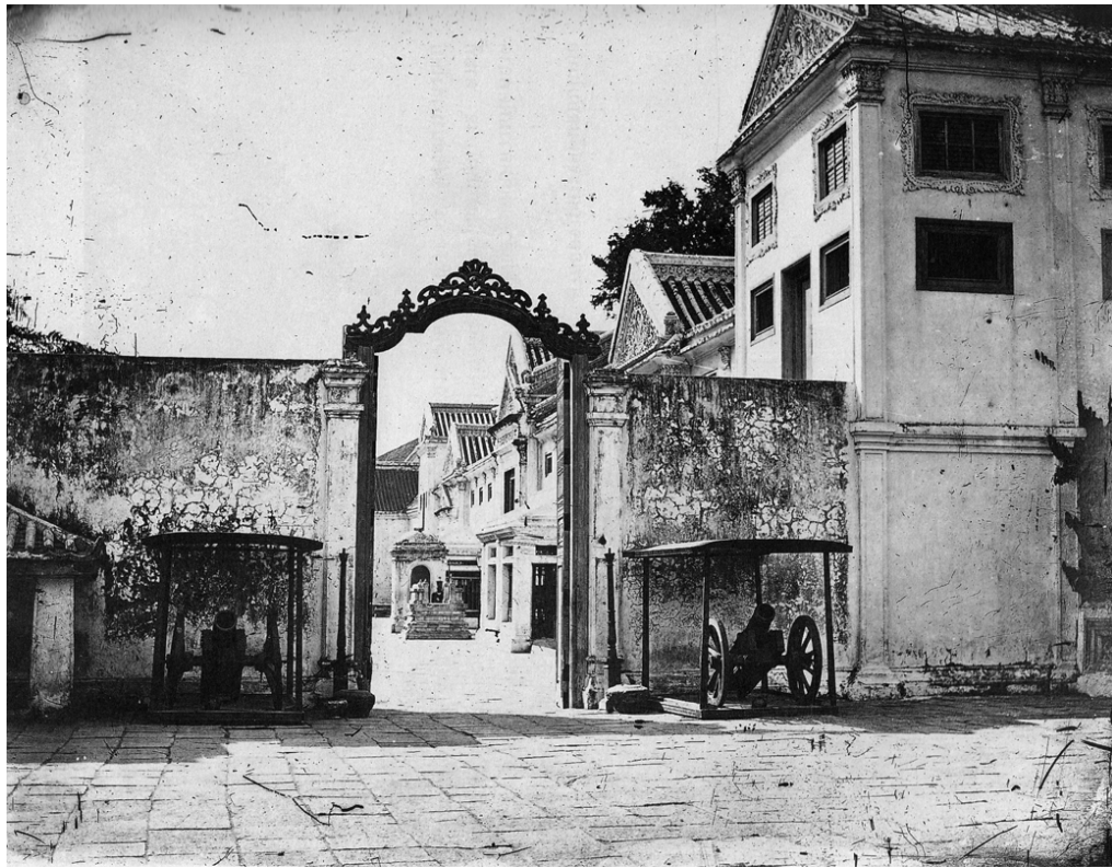
Figure 2.60 Entrance view, Phra Aphinaowaniwet. Source : NAT.
