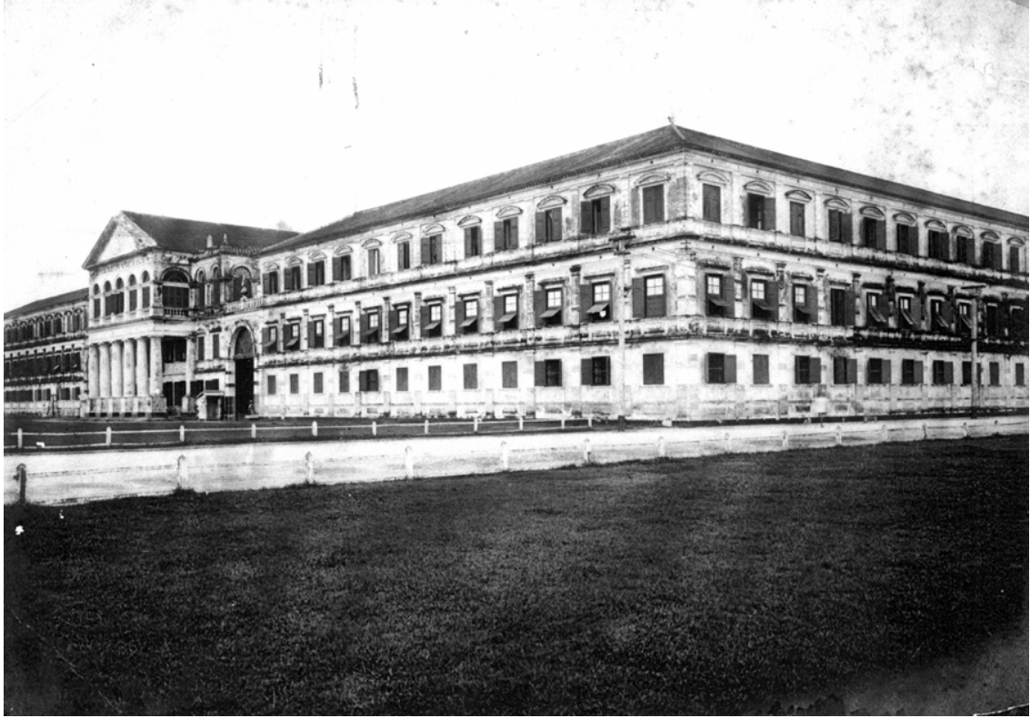
Figure 3.44 The Barracks (1881 – 1884). Source : NAT.
