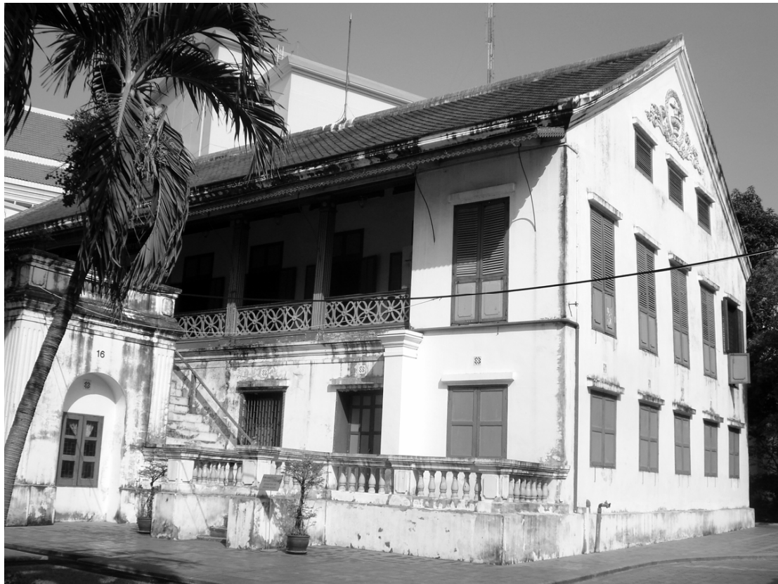
Figure 3.34 Itsaret Rachanuson Hall, Front Palace, Bangkok, an early Europeanized design by Siamese royal master builder, That Hongsakul. Source : Photograph by author.
