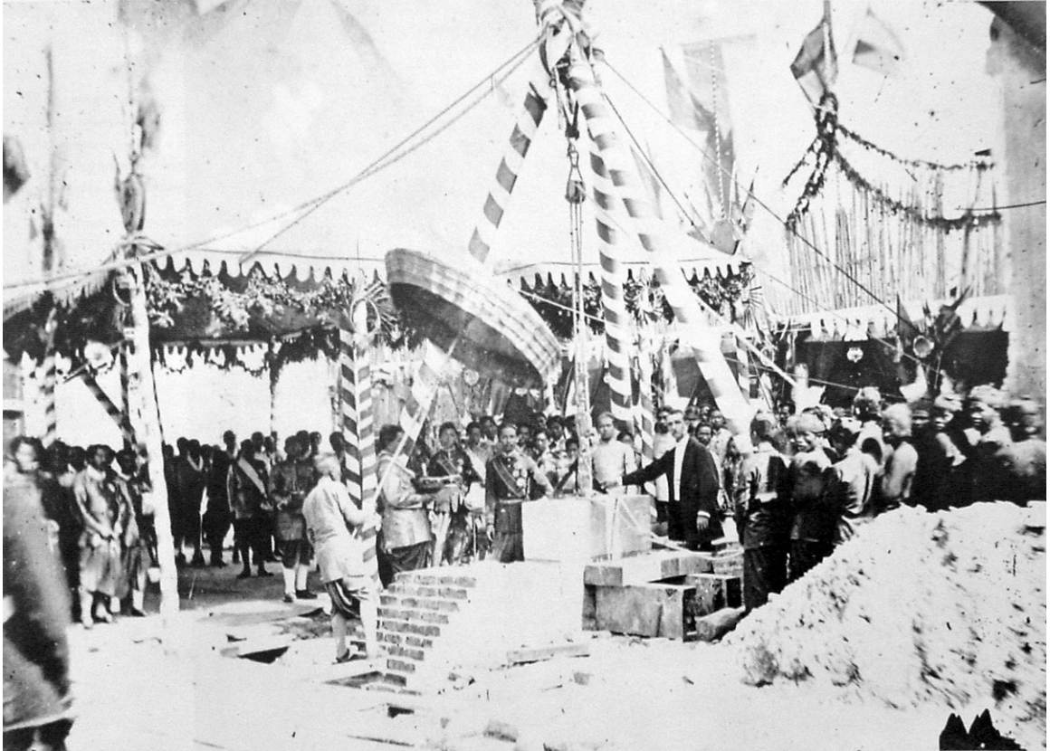
Figure 3.32 King Rama V (left, under the parasol) laying the foundation stone for the Chakri Throne Hall on May 17, 1876. John Clunis, Government Architect, stood to the right. Behind the king were the Siamese princes and noblemen, standing under a tent. Chinese and Siamese laborers stood to the right. Source : NAT.
