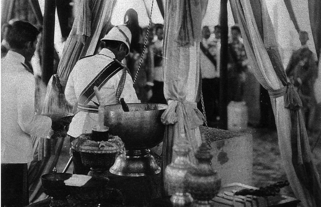
Figure 4.60 Rama V laying the foundation stone of Anantasamakhom Hall. Source : NAT.
