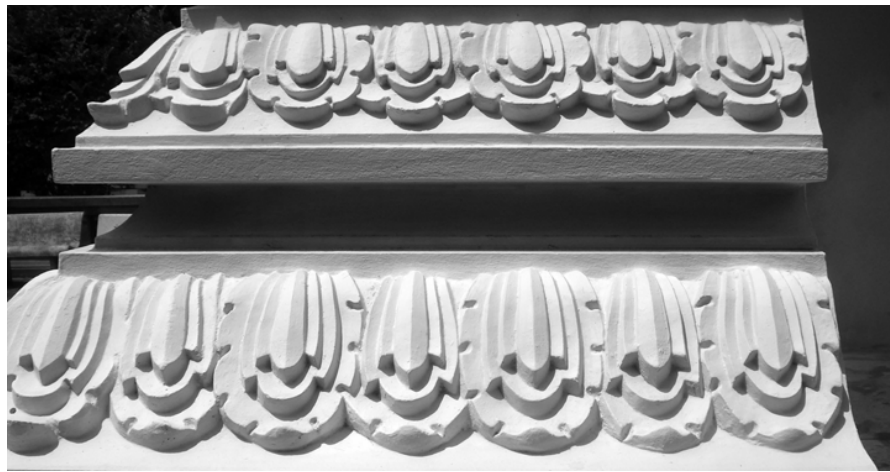
Figure 4.103 Precast-concrete detail, the ordination hall, Wat Rachathiwat.
