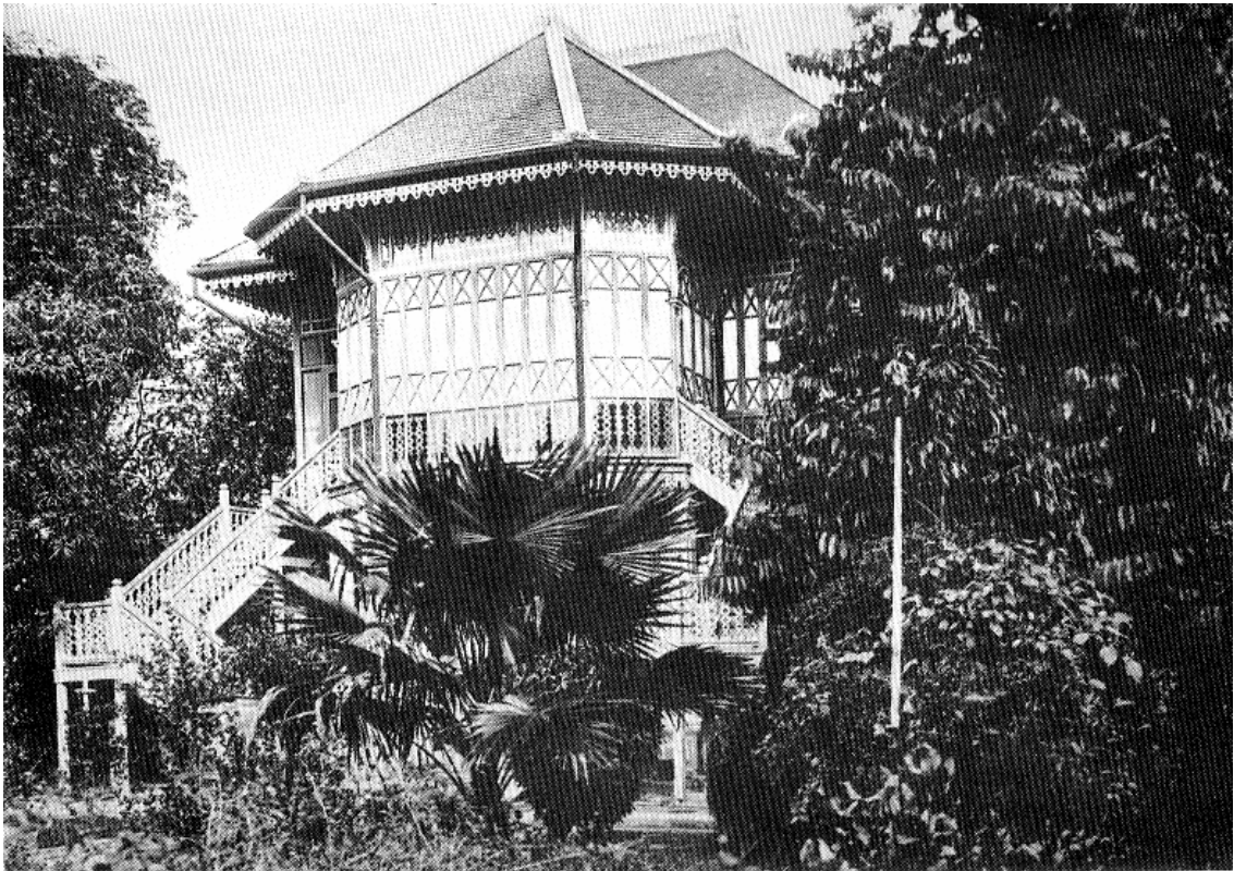
Figure 3.30 Victorian-style bungalow, Dusit Park Palace. Source : NAT.
