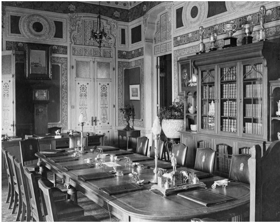
Figure 4.82 Council Chamber, Second Floor, Ambara Villa. Source : Malakul Family Album.
