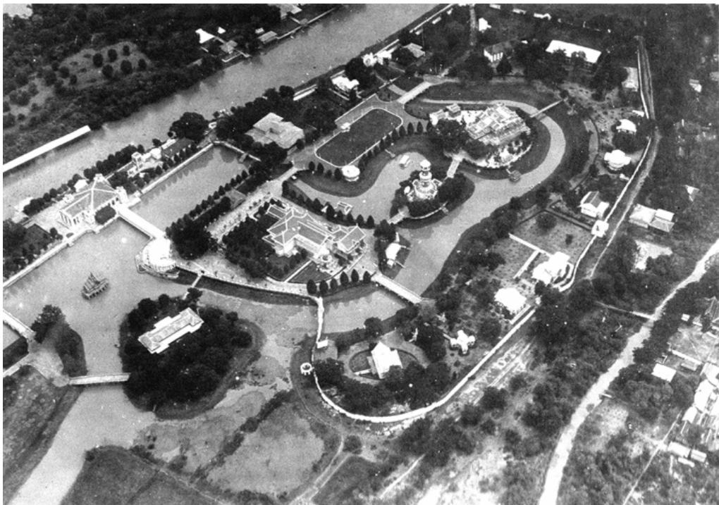
Figure 4.70 Aerial view of Bang Pa-In Palace, showing the king's residences surrounded by small bungalows and villas of the Inner Court. Source : NAT.
