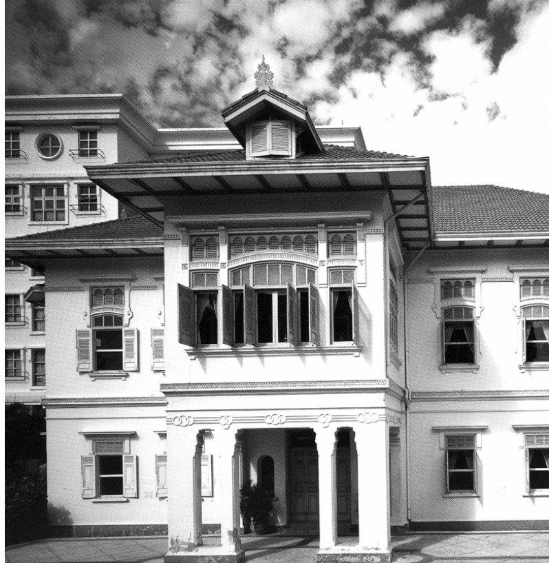
Figure 4.47 Dusit Park residence of Phraya Prasertsupphakit (Nop Krairoek), Rama V's butler. Source : ASA.
