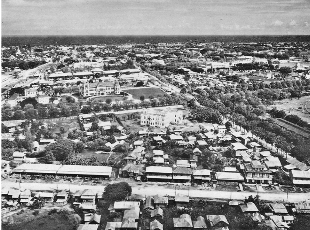
Figure 4.73 Aerial view of Prince Abhakara's Palace. The prince's residence occupied a corner of the triangular-shaped site, surrounded by fifteen houses for his wives. Source : NAT.
