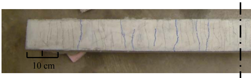
Figure 9 Experimentally observed surface cracking of ECC repair layer. This picture shows a half of ECC repair system. The blue marks indicate the cracks with the width between 40 µm and 60 µm, and the black marks indicate the cracks with the width smaller than 40 µm.
