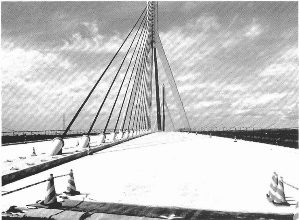
Figure 6: The Mihara bridge (Hokkaido, Japan) uses a steel/ECC composite deck (Courtesy, T. Kanda).
