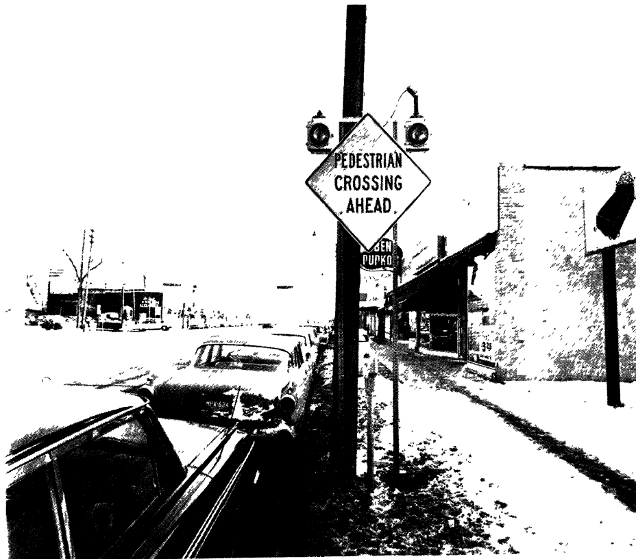
FIGURE 2-14 ADVANCE WARNING SIGN
