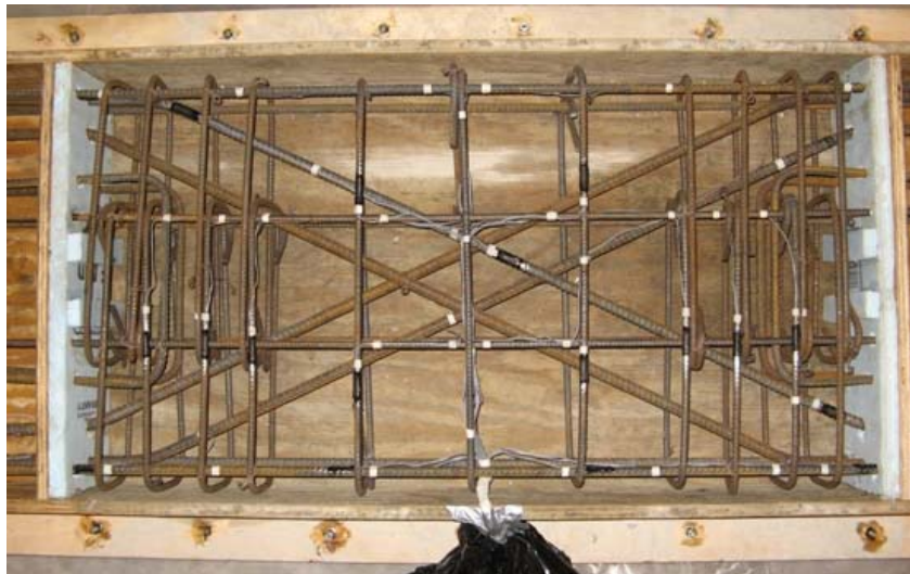
Figure 3.5 – Coupling beam reinforcement prior to casting HPFRC
