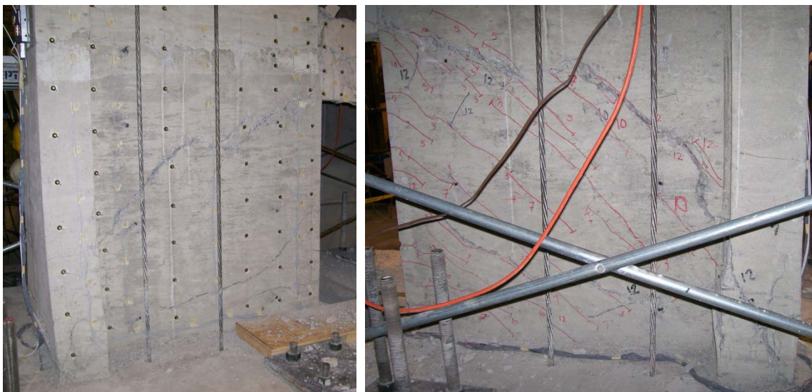
Figure 5.17 – Photographs of the failure plane in Specimen CW-2 from both faces of the wall specimen
