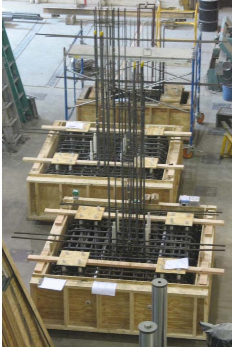
Figure 3.24 – Wall foundations prior to placement of concrete
