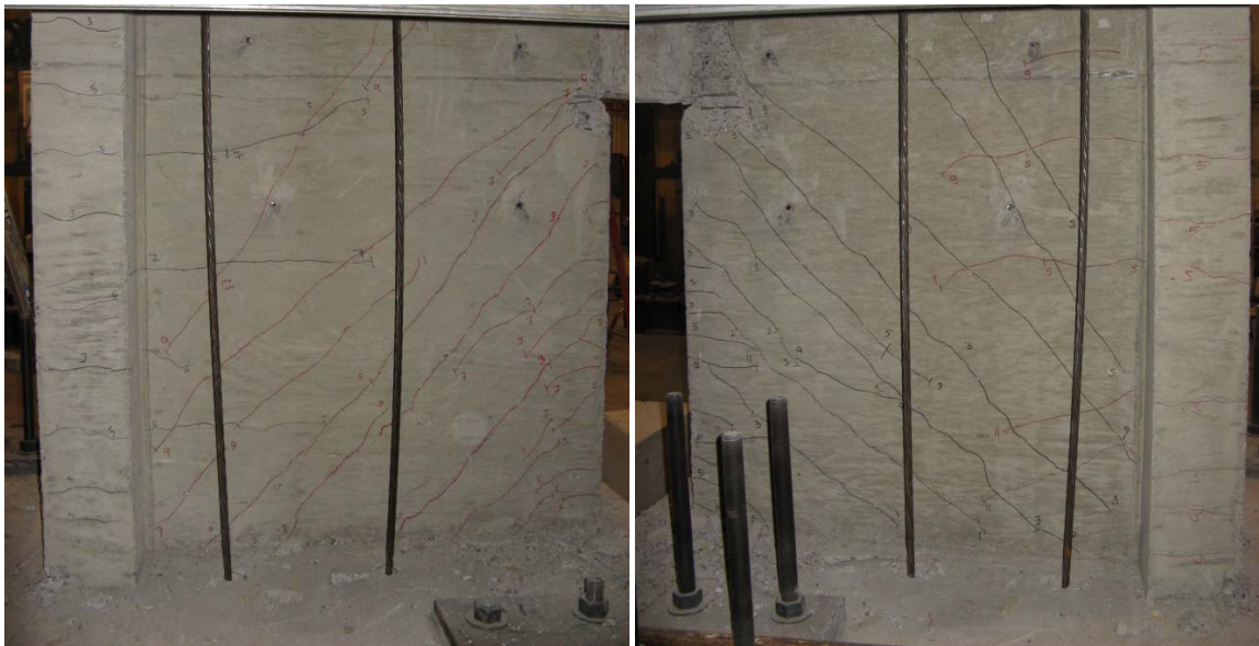
Figure 5.5 – Final damage state at the base of Specimen CW-1 (left and right are east and west walls, respectively). Diagonal cracks occurred when each wall was in compression; flexural cracks predominantly occurred while each wall was in tension.
