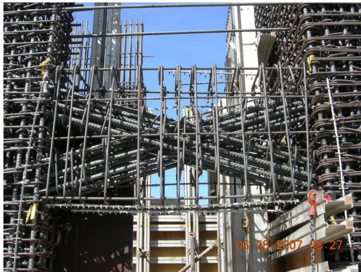
Figure 2.6 – On-site photo of diagonally reinforced coupling beam
