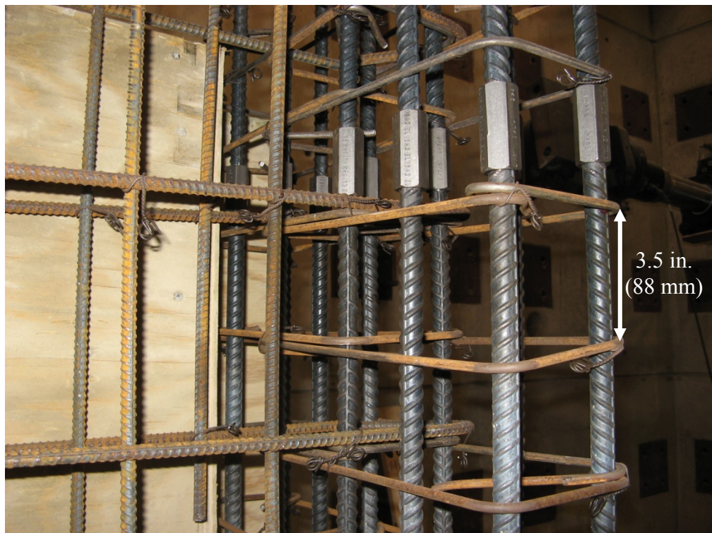
Figure 3.23 – Mechanical splice for #5 (D16) longitudinal reinforcement in walls
