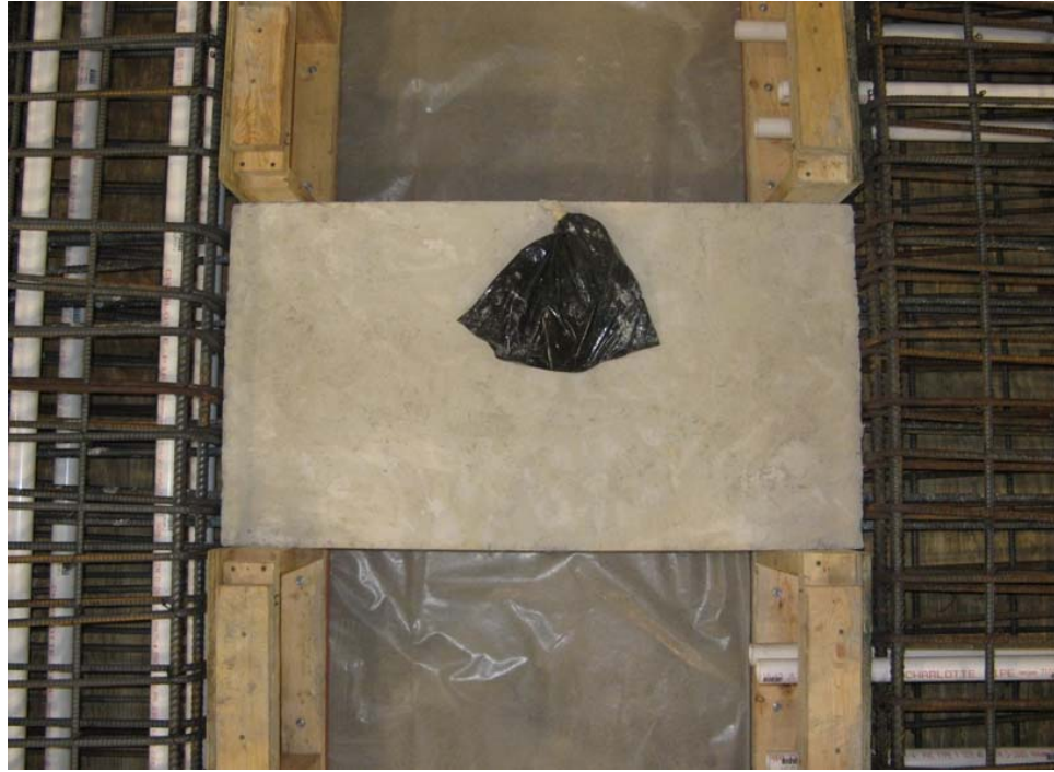
Figure 3.6 – Precast coupling beam prior to end block casting
