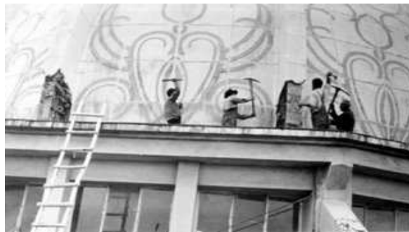
Figure 4. 2. The destruction of the dome of the National Baha'i Center.
