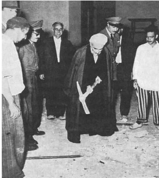
Figure 4. 4. Falsafi posing with a pickaxe as he takes part in the demolition.
