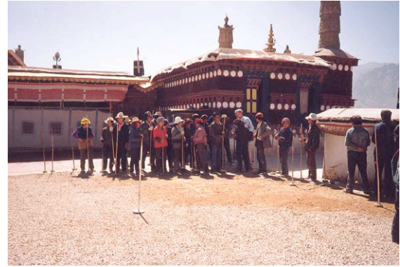
Tibetan peasants tamping down rocks on the roof of the Potala (with Ken and Bob)
