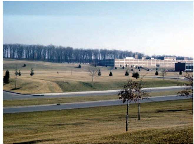
1970s Early construction on the North Campus
