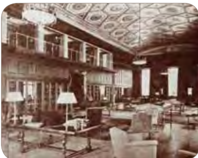
Main Reading Room
