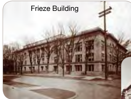
Frieze Building Addition
