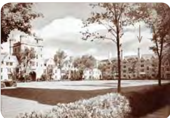
Dormitory Wing (left) John P. Cook Wing (right)
