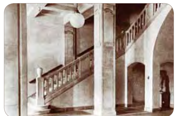
Lorch Hall Entrance Lobby
