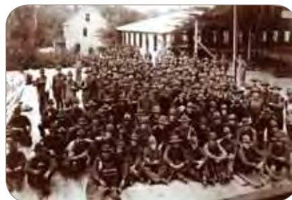
Building a Temporary Mess beside the Michigan Union
