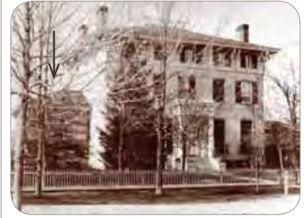
In 1864 the Havens added the one-story kitchen (left).
