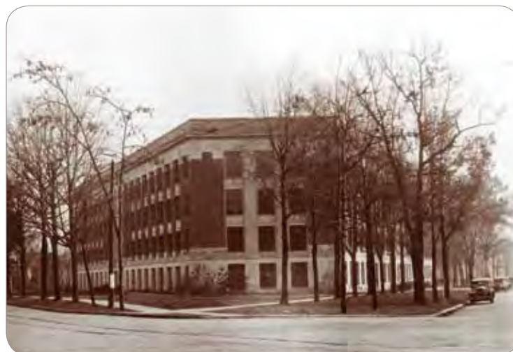
East Medical Building
