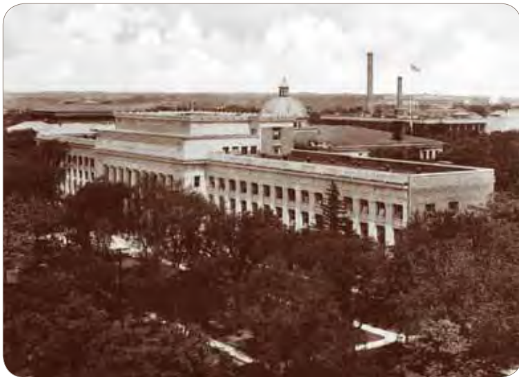
Only the middle section of the original plan was constructed.
