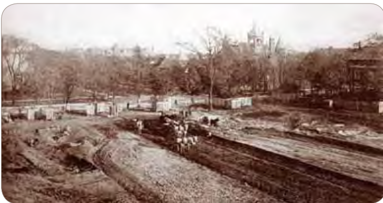
Excavation for the New Michigan Union
