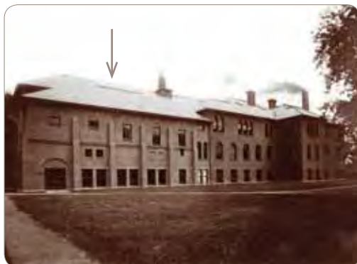
Physics Laboratory Addition (left)
