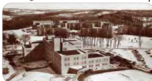
Women s Hospital (front) University Terrace Apartments (rear)
