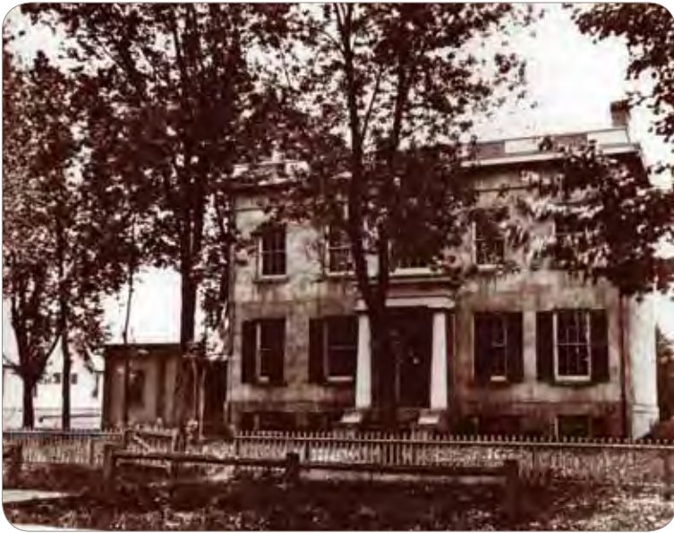
Original Professors House (facing street)
