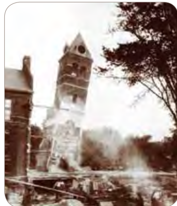
Demolition of the University Library Tower, July, 1917
