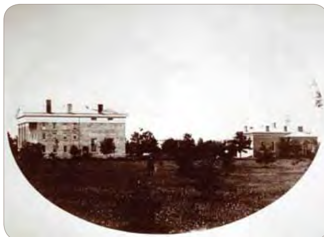
Medical Building (left), Chemical Laboratory (right)
