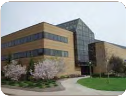
The FXB Building
