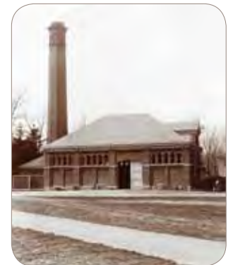
Heating Plant Behind University Hall
