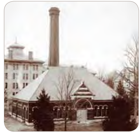
Heating Plant - Medical Building (rear)
