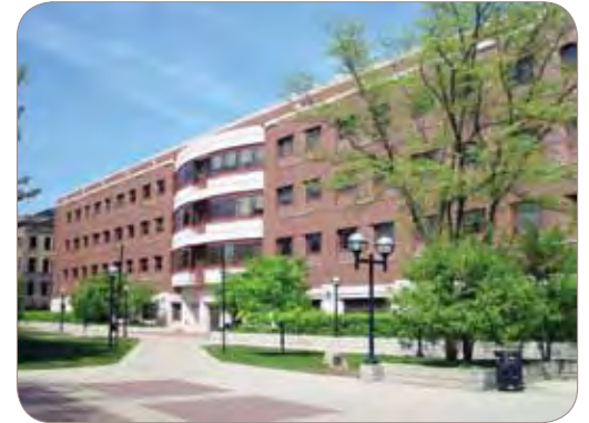
Randall Physics Addition
