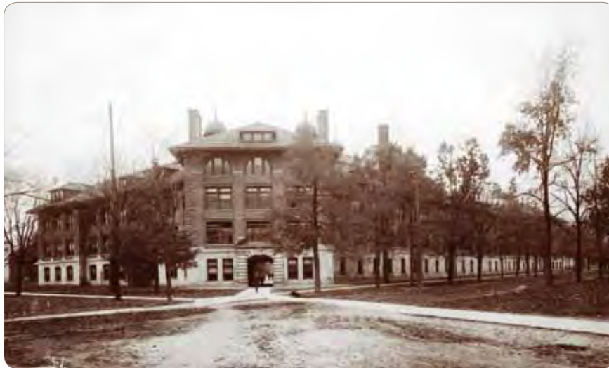
The New Engineering Building
