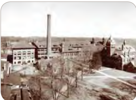
West Engineering, Engineering Shops Old Heating Plant
