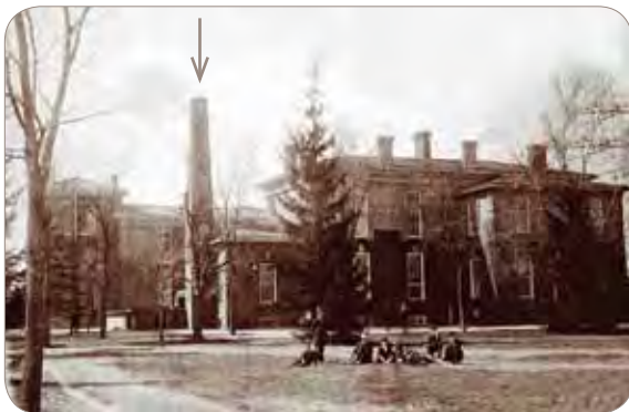
Heating Plant East End of the Chemical Laboratory
