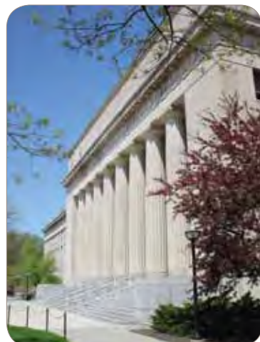
Angell Hall Renovation
