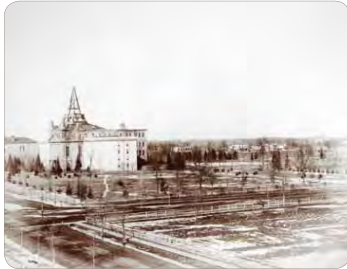
University Hall under Construction Completed in 1872
