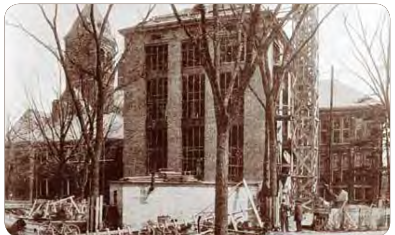
Stacks Being Built around the Old Library
