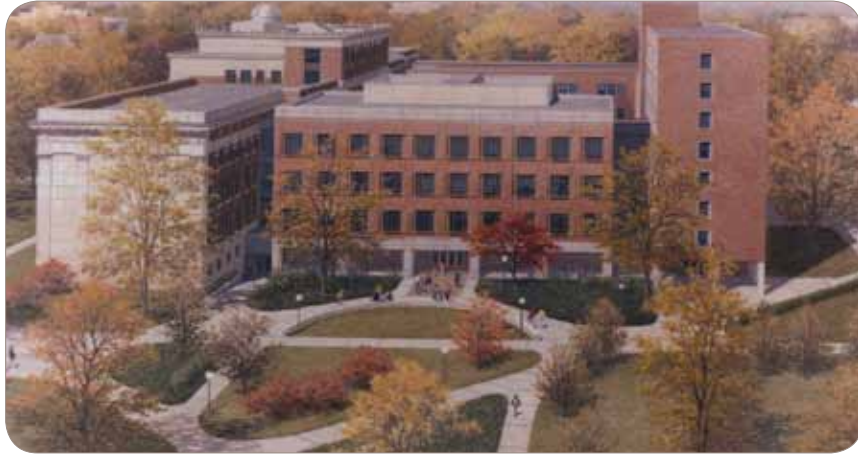
Tisch Hall - Angell/Haven Addition
