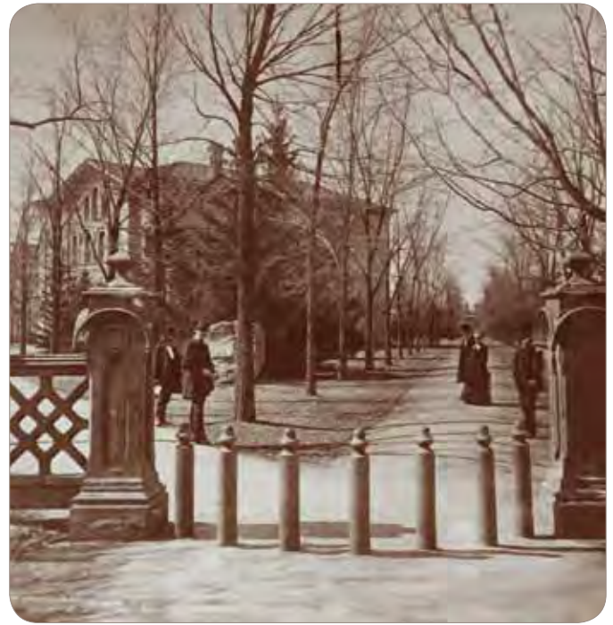
Fence with Posts
