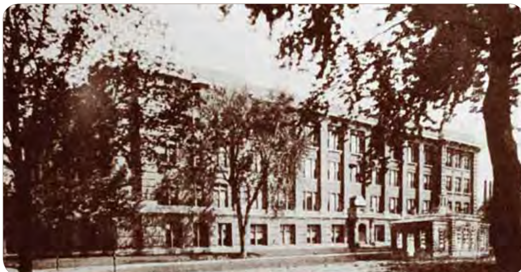
The New Chemistry and Pharmacy Building (The original Chemical Laboratory is inset at lower right.)
