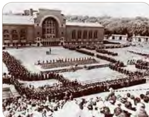
Commencement at Ferry Field
