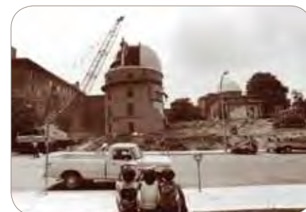
Demolition of the old Astronomy Building
