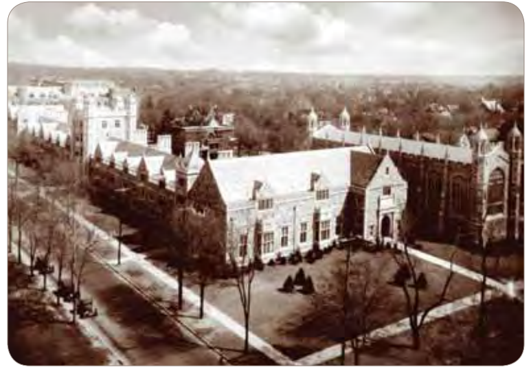
Dormitory Wing, Lawyers Club and Dining Hall
