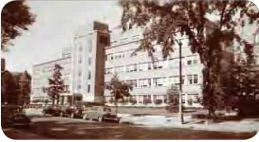
Administration Building on State Street
