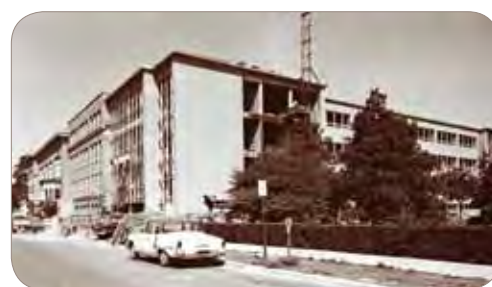
Frieze Building Addition 1957
