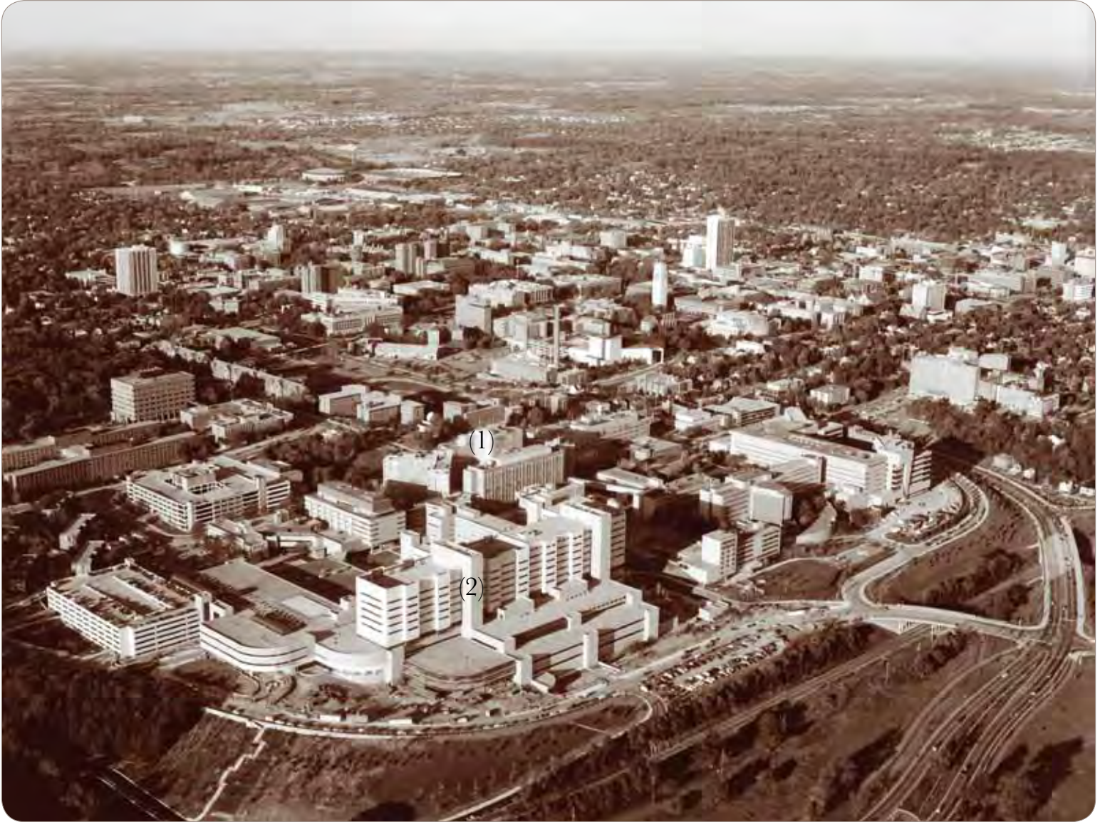
Old Main Hospital (1) Replacement Hospital (2)
