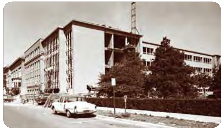
Frieze Building Addition 1957
