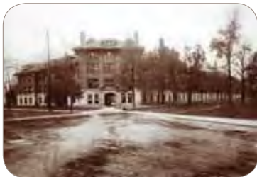
New Engineering Building
