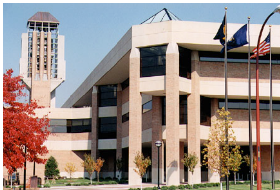
The Millennium Project in the University of Michigan Media Union
