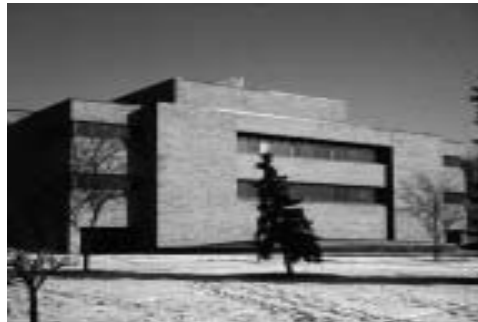
Herbert H. Dow Building Media Center Renovations June, 1986 Architect: Simms-Varner Contractor: Fairview Construction Cost: $3,016,347
