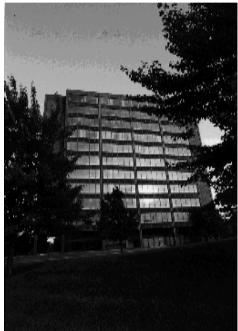
Wolverine Tower Renovations Phase I & Phase II June 1994 Architect: Rossetti Architects Contractor: J. C. Beal Construction Cost: $2,094,784
