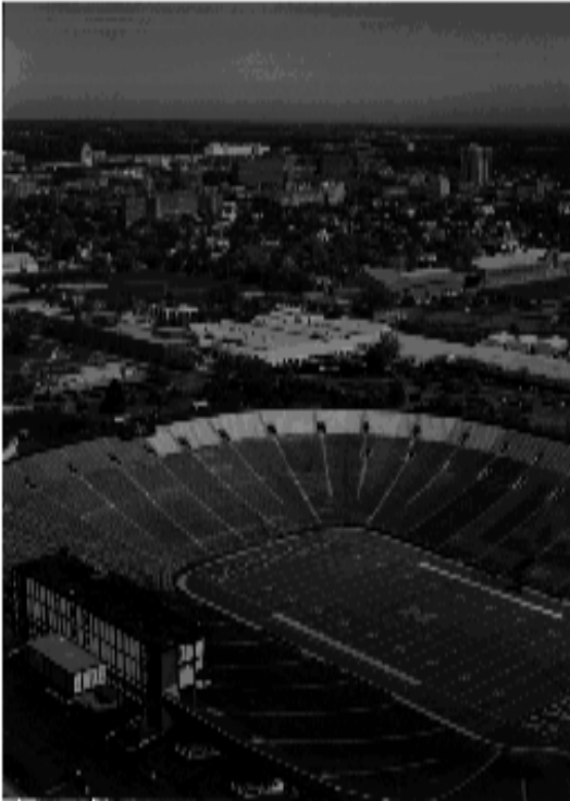
University of Michigan Football Stadium Prescription Turf February 1993 Architect: Luckenbach/Ziegelman & Partners Contractor: Turf Services, Inc. Cost: $2,164,303
