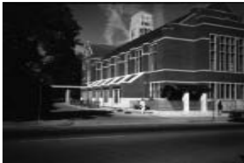
Michigan League Renovation & Addition December 1987 Architect: Fry & Associates Contractor: TKI Construction Management Cost: $1,100,000
