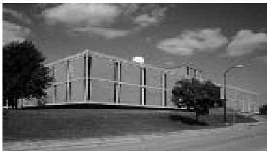
Space Research Laboratory Addition - East Side May 1992 Architect: UM Facilities Planning & Design Contractor: John M. Olson Company Cost: $2,715,322
