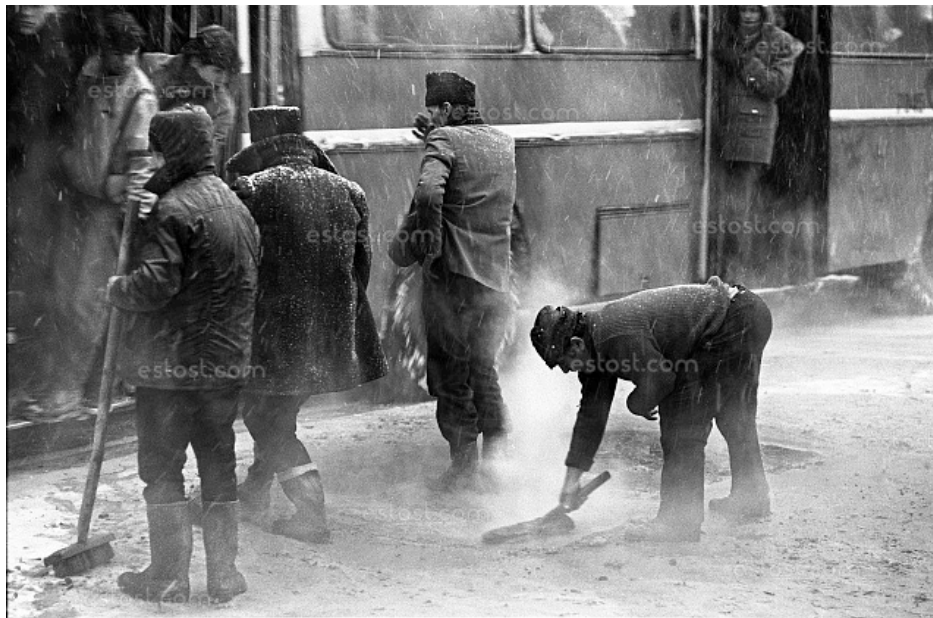
Fig. 9: Pouring new cement in heavy sleet, Bucharest, 1985. 205
