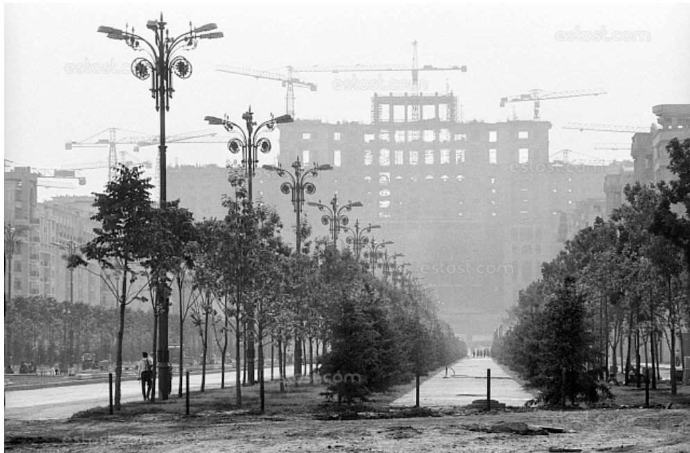
Fig. 10: The Palace of the People during construction. The Romanian army guards the site with Kalashnikovs, Bucharest, 1986. 207
