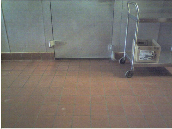
Photo 38 - Refrigerator Exterior Door in Kitchen of YCC Facility
