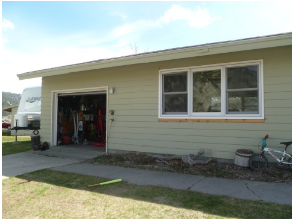
Photo 16 - Front, Exterior of Residence
