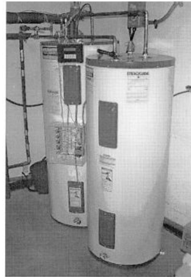
Photo 90 - Hot Water Storage Tank 101
