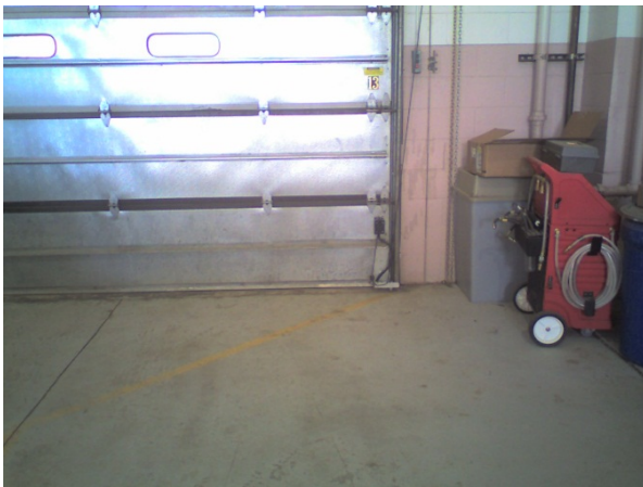
Photo 28 - Lower Interior High Bay Garage Door
