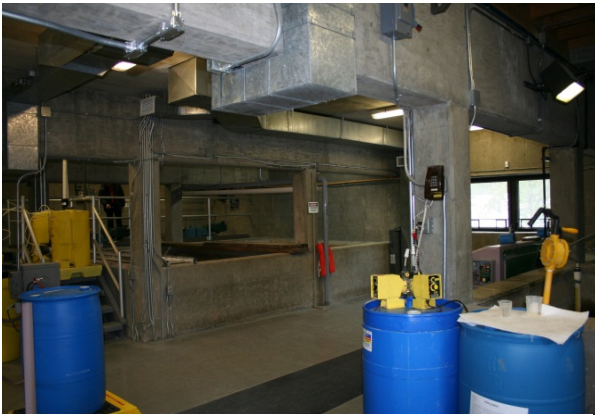
Photo 78 - Old Faithful Water Treatment Plant
