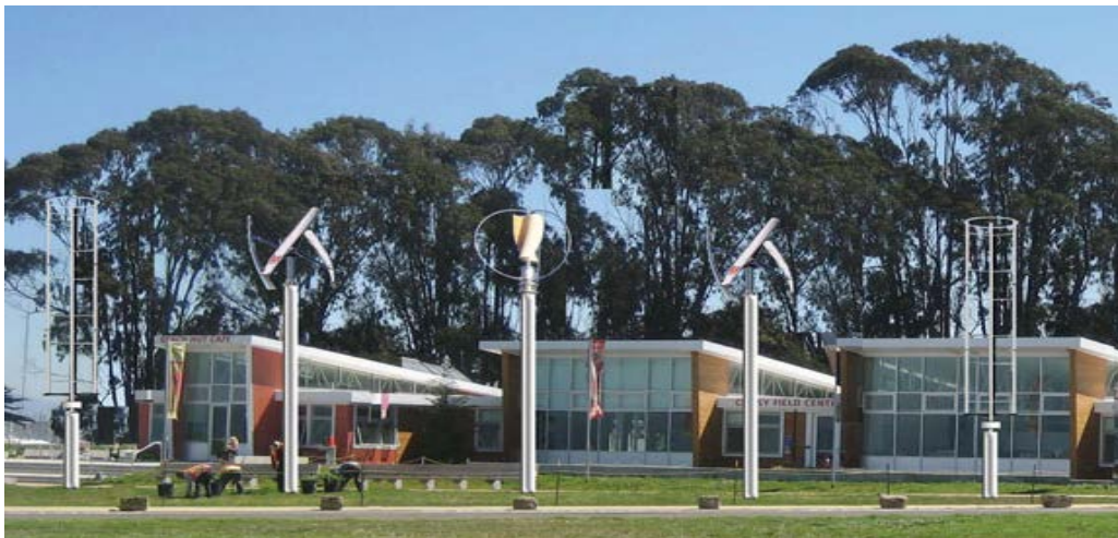
Photo 92 - Wind Turbine Installation at Crissy Field 106
