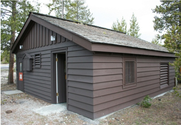
Photo 76 - Old Faithful Inn Lift Station
