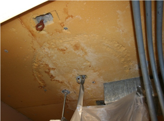
Photo 77 - Old Faithful Main Lift Station
