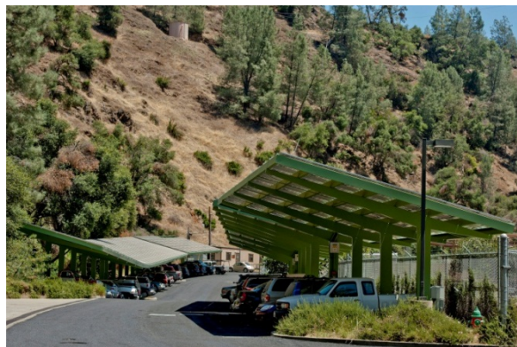
Photo 88 - Parking Lot Canopies at Yosemite Equipped With Solar Arrays 99
