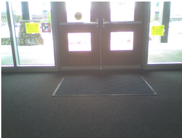
Photo 56 - Main Exterior Doors
