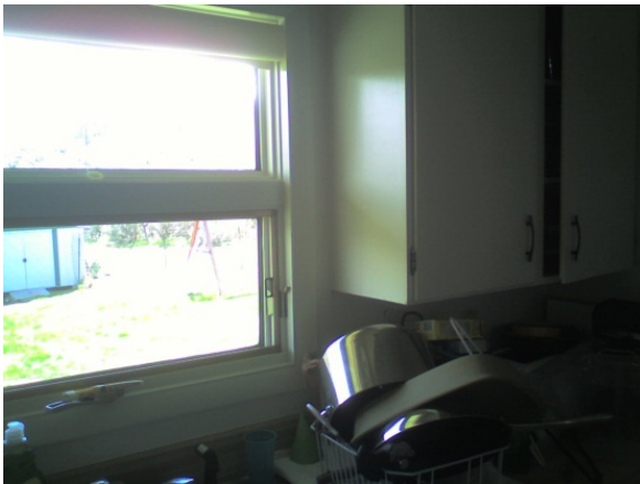
Photo 18 -Missing Insulation Strip Between Window and Cabinet
