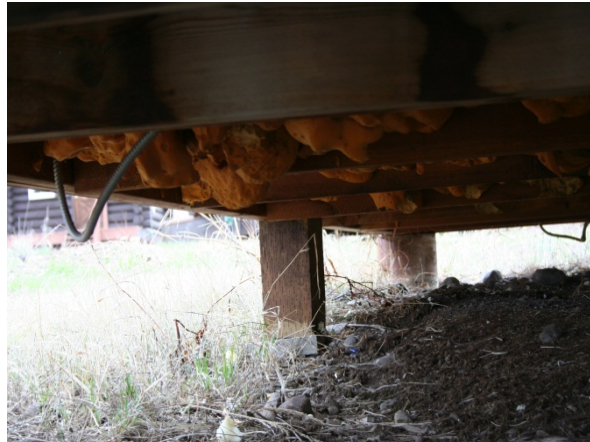
Photo 72 - Bottom of a YA Cabin
