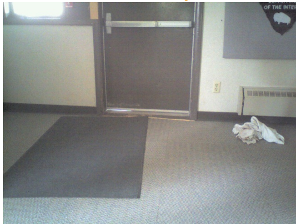
Photo 40 - Exterior Door Facing Dorms
