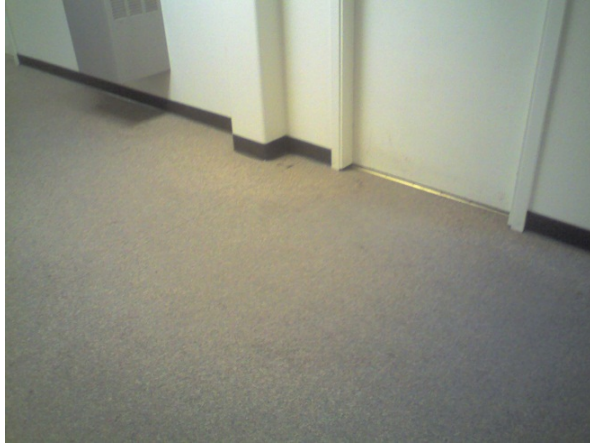
Photo 32 - Floor Near Water Fountain
