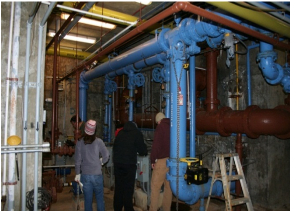
Photo 79 - Old Faithful Water Treatment Plant
