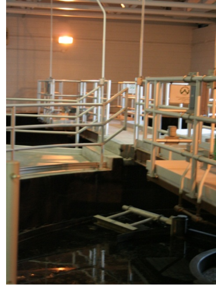
Photo 82 - Canyon Waste Water Treatment Plant
