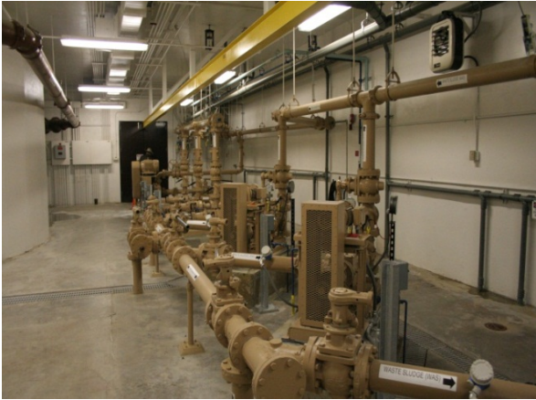
Photo 81 - Canyon Waste Water Treatment Plant
