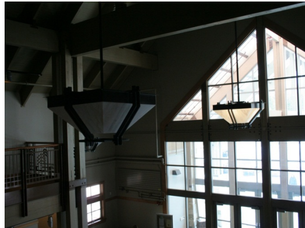
Photo 62 - Light Turned on Near Windows
