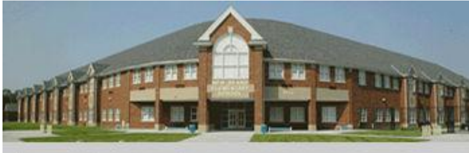
(New James Beard Elementary; J. L. Judge Construction Services Company, LLC, 2009)
