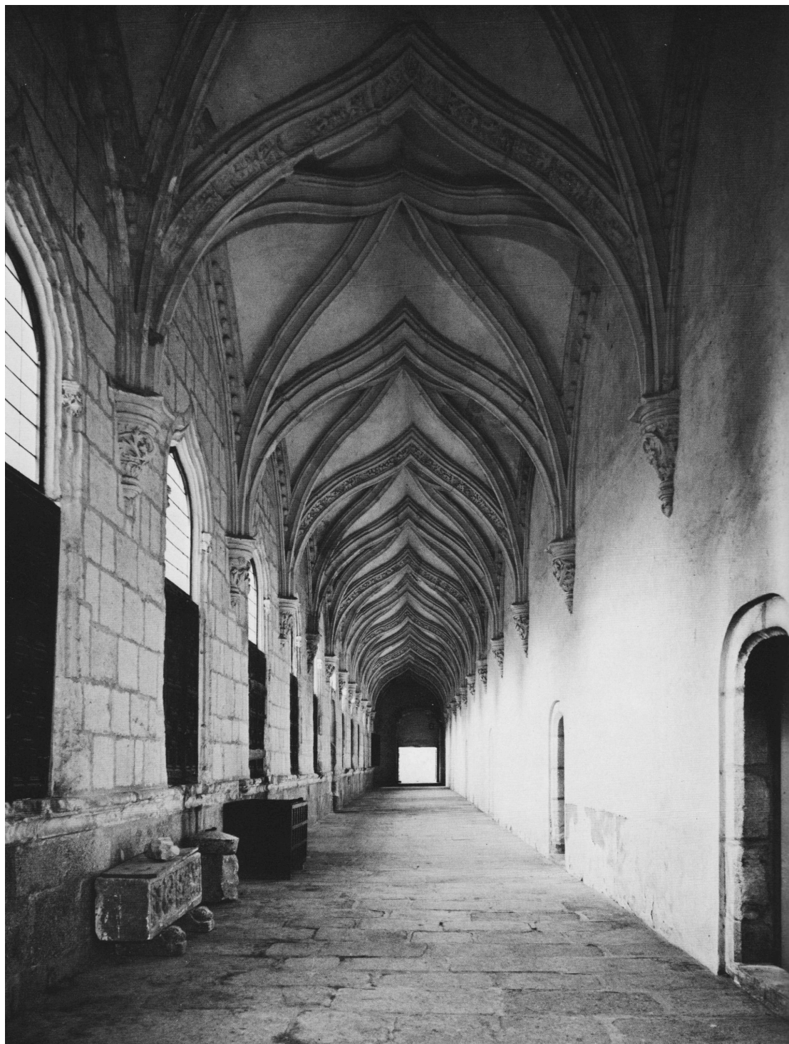
Figure 3.23. Charterhouse of El Paular, monks' cloister, east alley. Photo: Gómez, La Cartuja , fig. 36.
