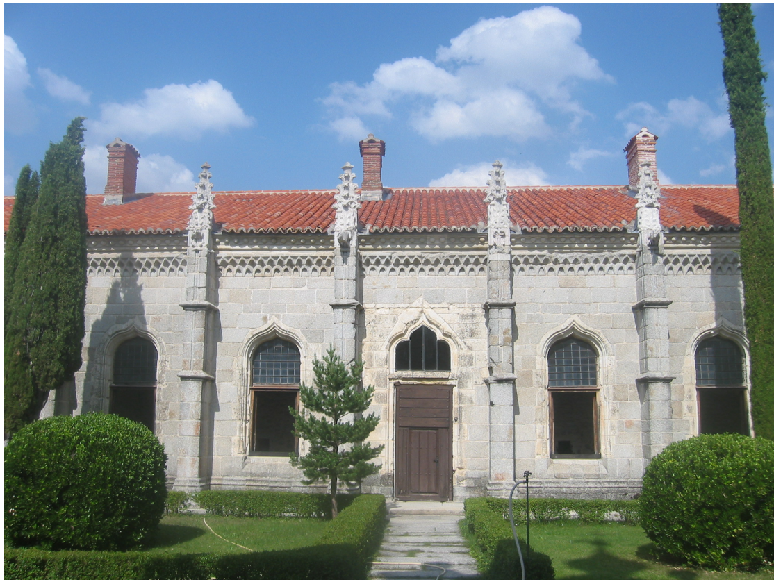
Figure 3.73. Charterhouse of El Paular, exterior of monks' cloister.
