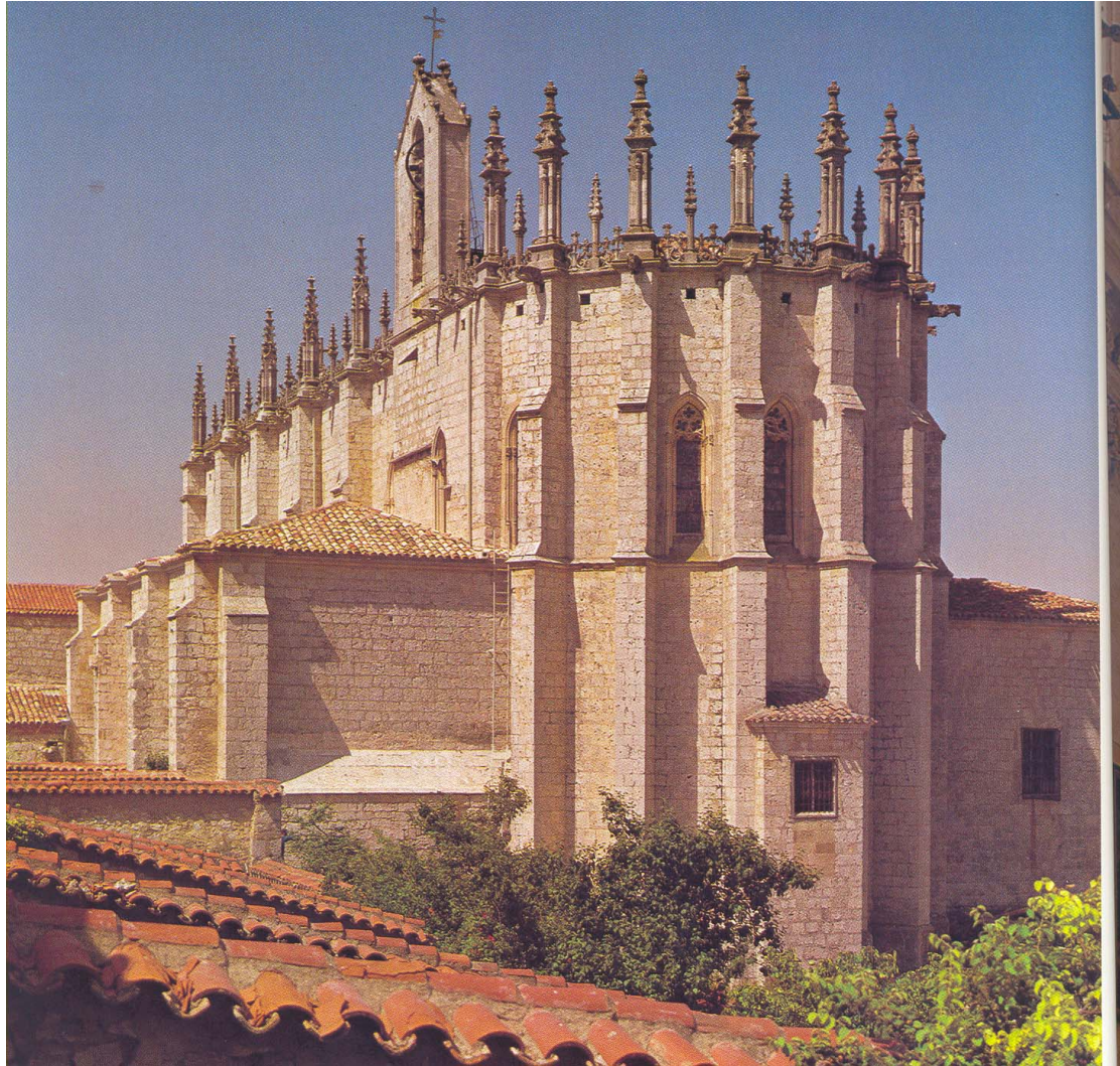
Figure 3.50. Charterhouse of Miraflores, exterior of church showing ashlar masonry and pinnacles. Photo: MC4:2 , fig. 58.
