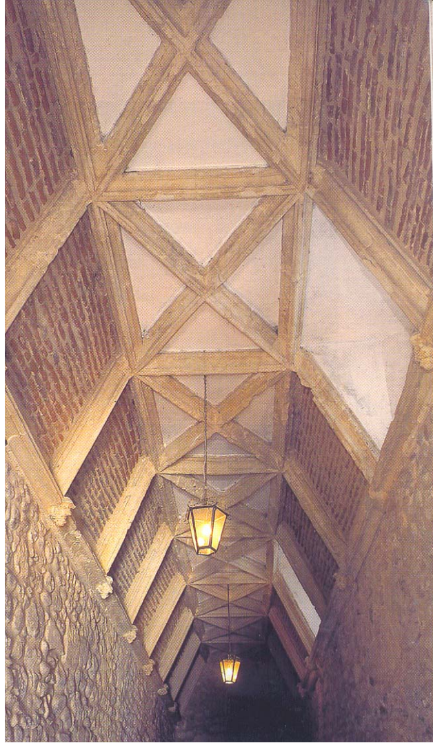
Figure 3.18. Charterhouse of El Paular, hallway between covered porch and monks' cloister.
