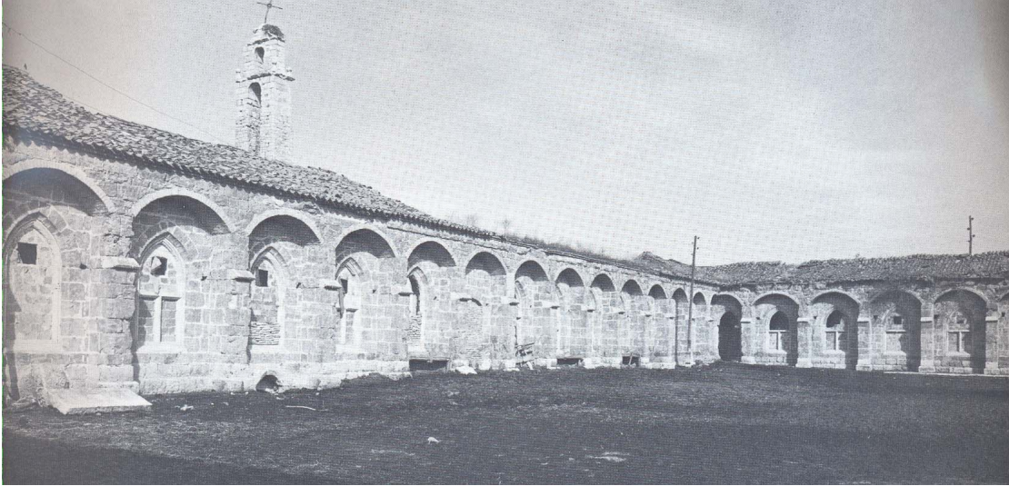
Figure 3.69. Charterhouse of Aniago, cloister.
