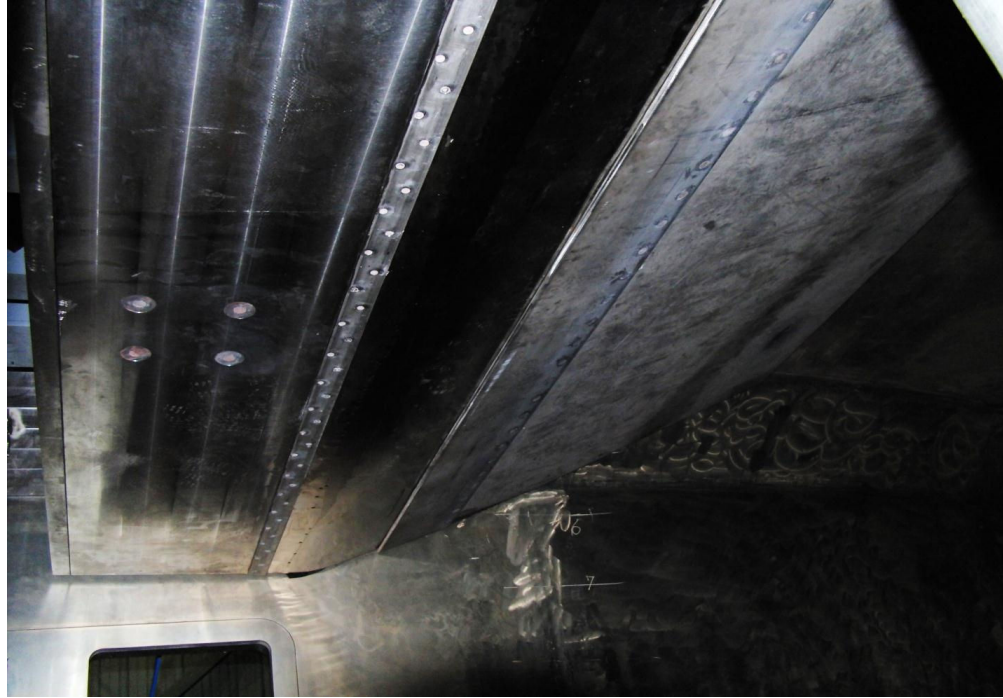
Figure A.16 – Gate in the test section with the flap at 0 degrees with respect to the horizon. The gate's hinge was covered by a flexible spring steel sheet which slid in and out of the slot upstream, always providing a smooth flow surface and minimizing water leakage through the hinge.
