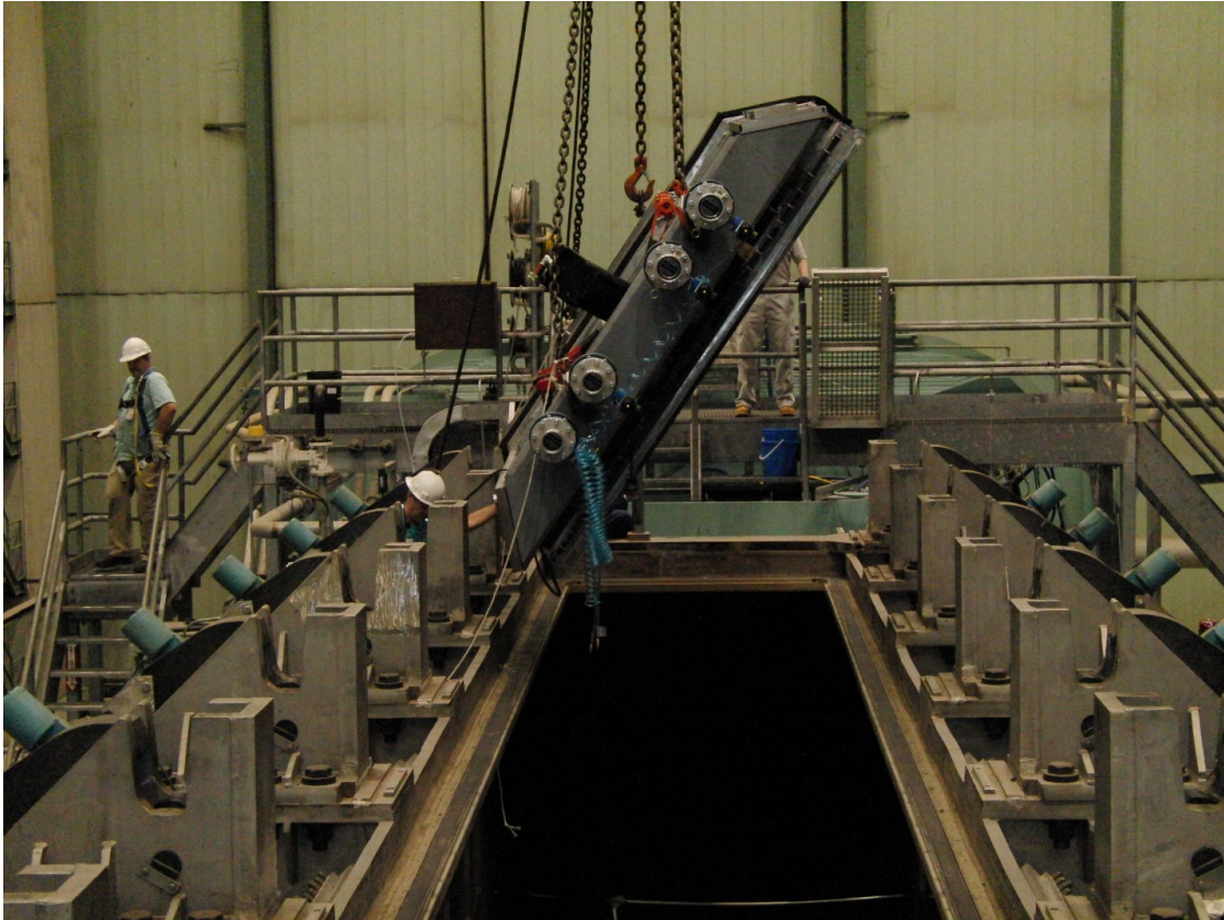
Figure A.15 – To get the gate into the test section it had to be tilted by over 45 degrees. Once in the test section, it was lowered onto a cart and the crane disconnected so that the chains could be repositioned for the final lift into position, during which the chains upstream went through the window on the LCC’s ceiling upstream of the test section.
