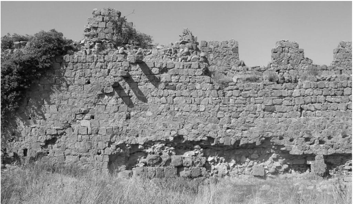
Figure A2.12: Remains of Etruscan city-wall blocks (below) built into the medieval city wall at Cencelle.
