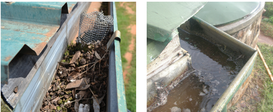
Figure 63: Poorly maintained gutters at MRC, August 2011
