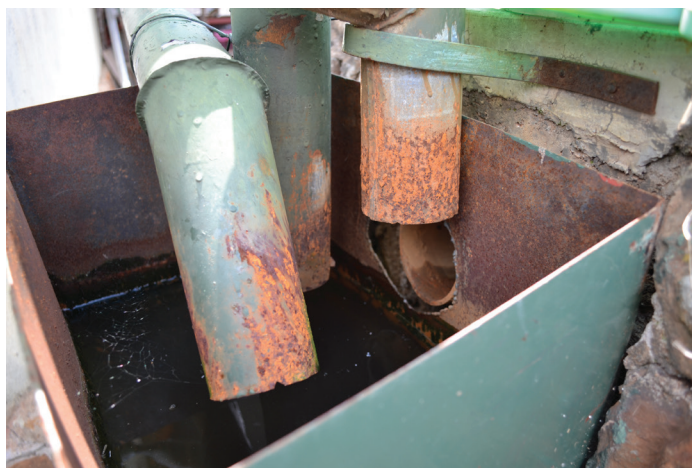
Figure 64: Disconnected storage infrastructure at McCormack Lab, August 2011
