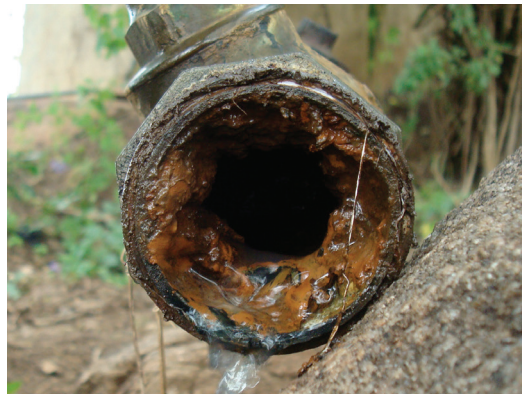
Figure 57: Photograph of a pipe interior at Mpala
