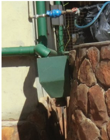
Figure 65: Repaired rainwater harvesting system at McCormack Lab, March 2012
