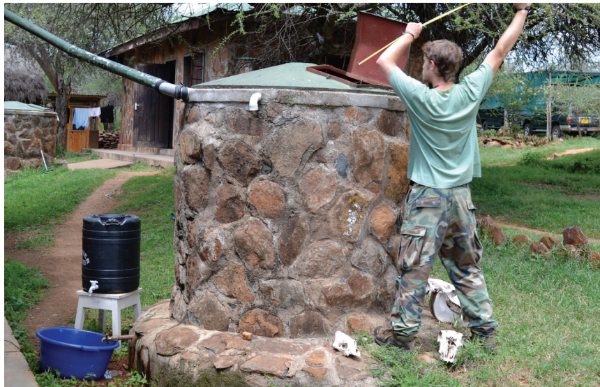
Figure 41: Kitchen rainwater harvesting tank
