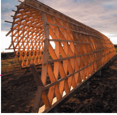
Figure 1.68: Example of a completed lamella structure
