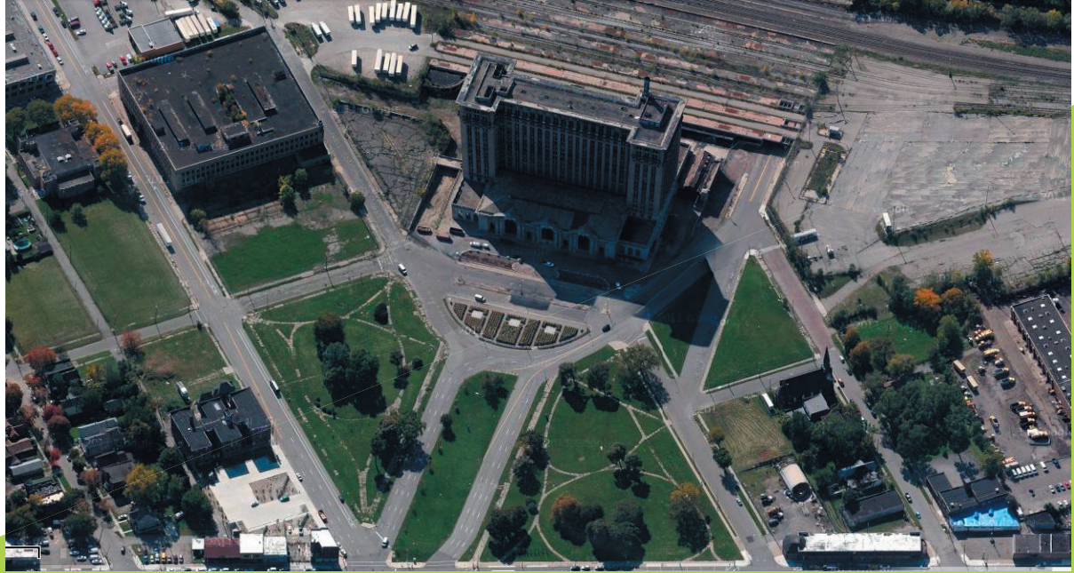
Figure 2.29 (below): the Roosevelt Park site existing conditions from above
