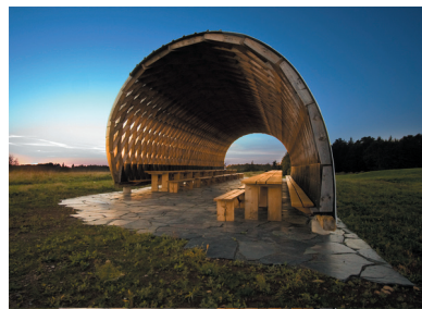
Figures 2.18 (above) + 2.19 (right) + 2.20 (far right): Example of a lamella structure built by the Coastal Studio
