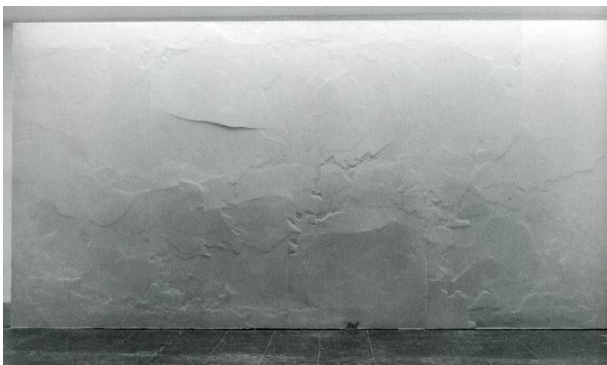
Fig. 22 Shmueli’s wall (detail 1)
