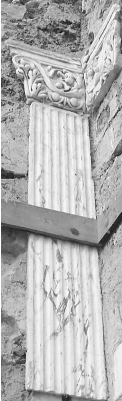
5.19. Detail of capital from pilaster zone in marble hall 2/31. Photo: author.
