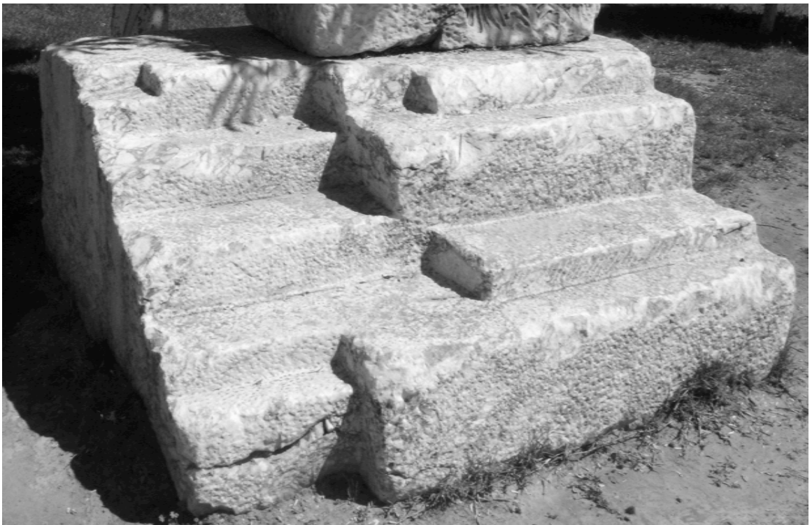
4.15. Block with stepped surface, intended as revetment. Photo: author.
