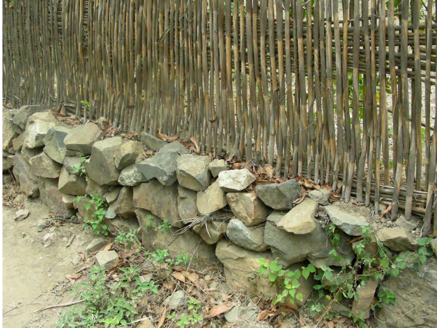
Figure 4.69. The wall of a modern house near Las Varas. Canes with stone foundation.
