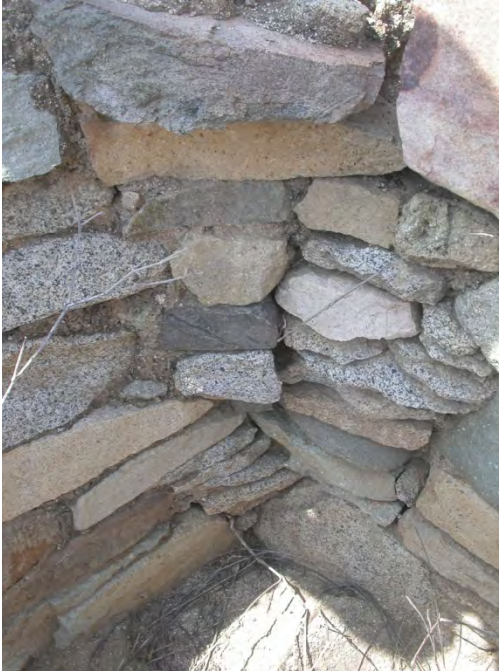
Figure 5.45. Cist Tomb 1 of Las Varas, showing details of construction.
