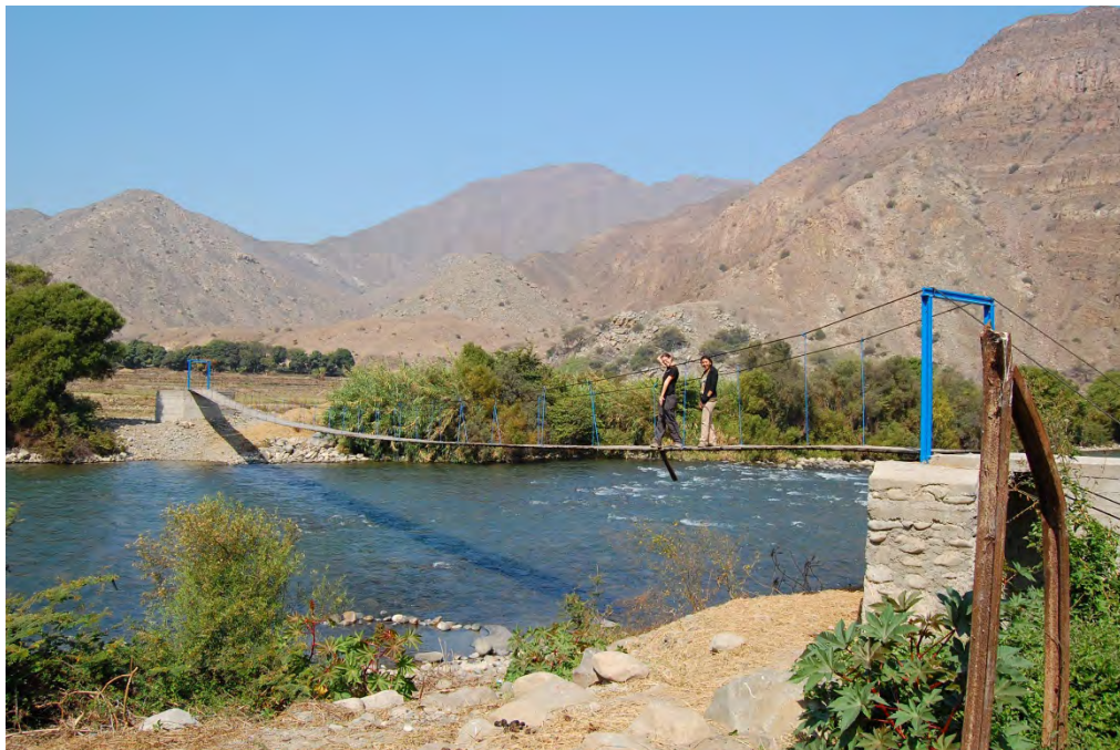
Figure 6.12. Robyn Cutright and Maritza Bazán standing on a bridge across the Jequetepeque River. The bridge was built in 2010, replacing the oroya .
