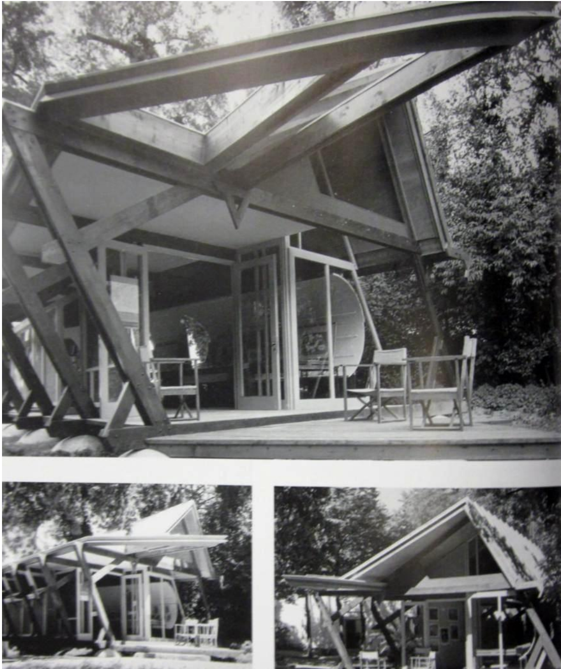
Figure 62. Carlo Scarpa, Il padiglione del libro (Book Pavilion), grounds of the Venice Biennale, Venice, Italy.
