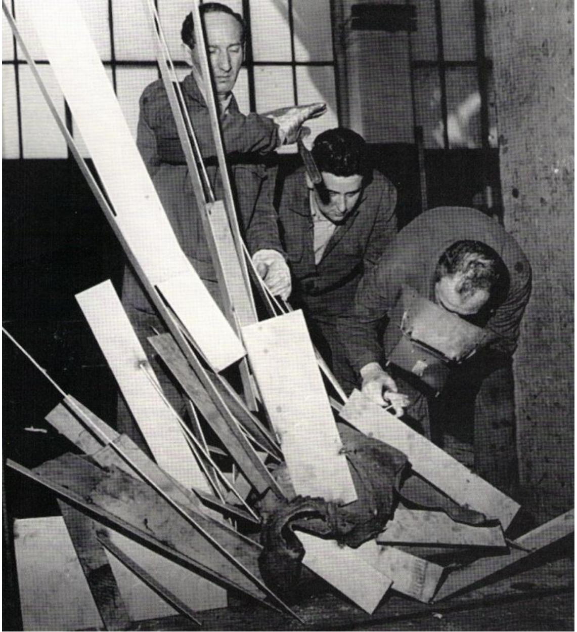
Figure 10. Eugenio Carmi working at Italsider di Cornigliano, 1962. Photograph by Ugo Mulas.
