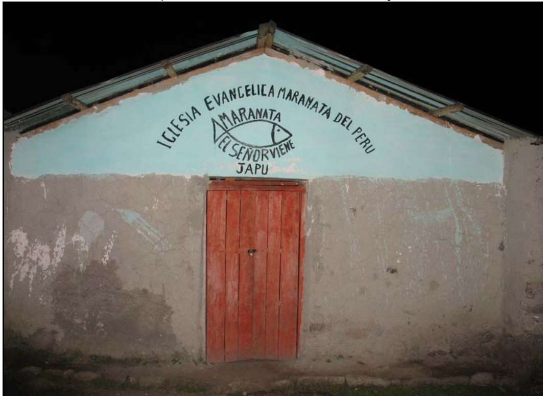
Figure 7.1 Façade of the Maranata Church in Hatun Hapu
