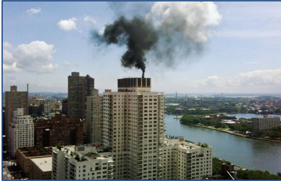
Figure 17. Soot Pollution Emitted From Number 4 and Number 6 Heating Oil Combustion in NYC.
