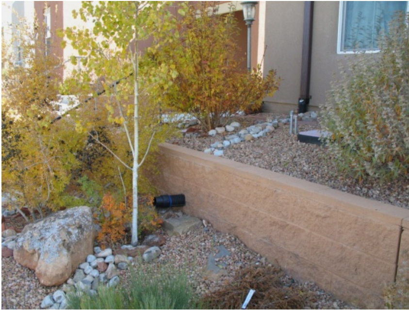
Image 4.7 La Entrada Downspout Drainage System
