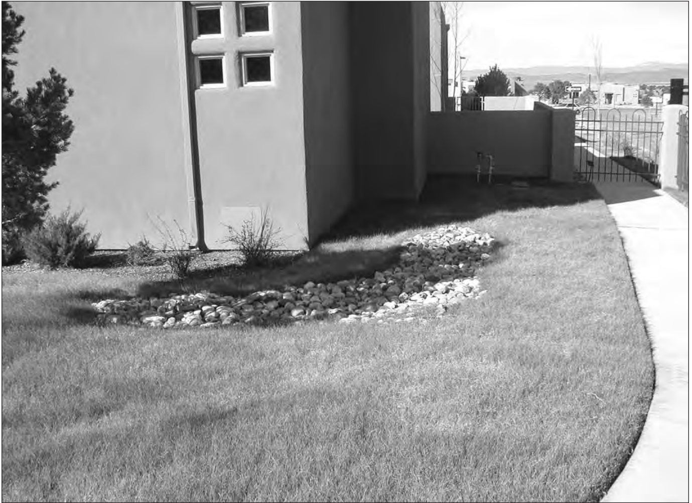
WATER-HARVESTING SYSTEM - COBBLE DRAINAGE WAY IN LAWN AREA WINDMILL RIDGE UNIT 1 - MODEL HOME VISTA SERIES
