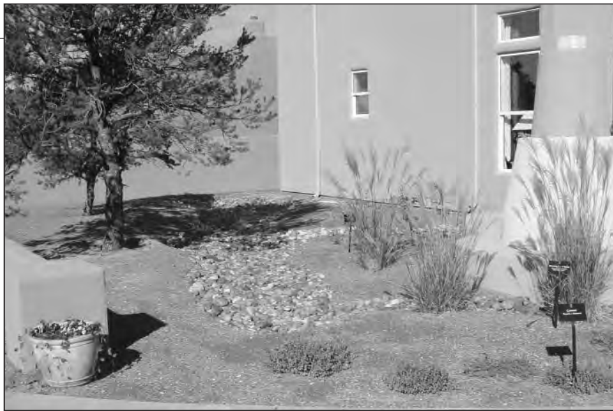
COBBLE DRAINAGE WAY IN CRUSHED STONE YARD
