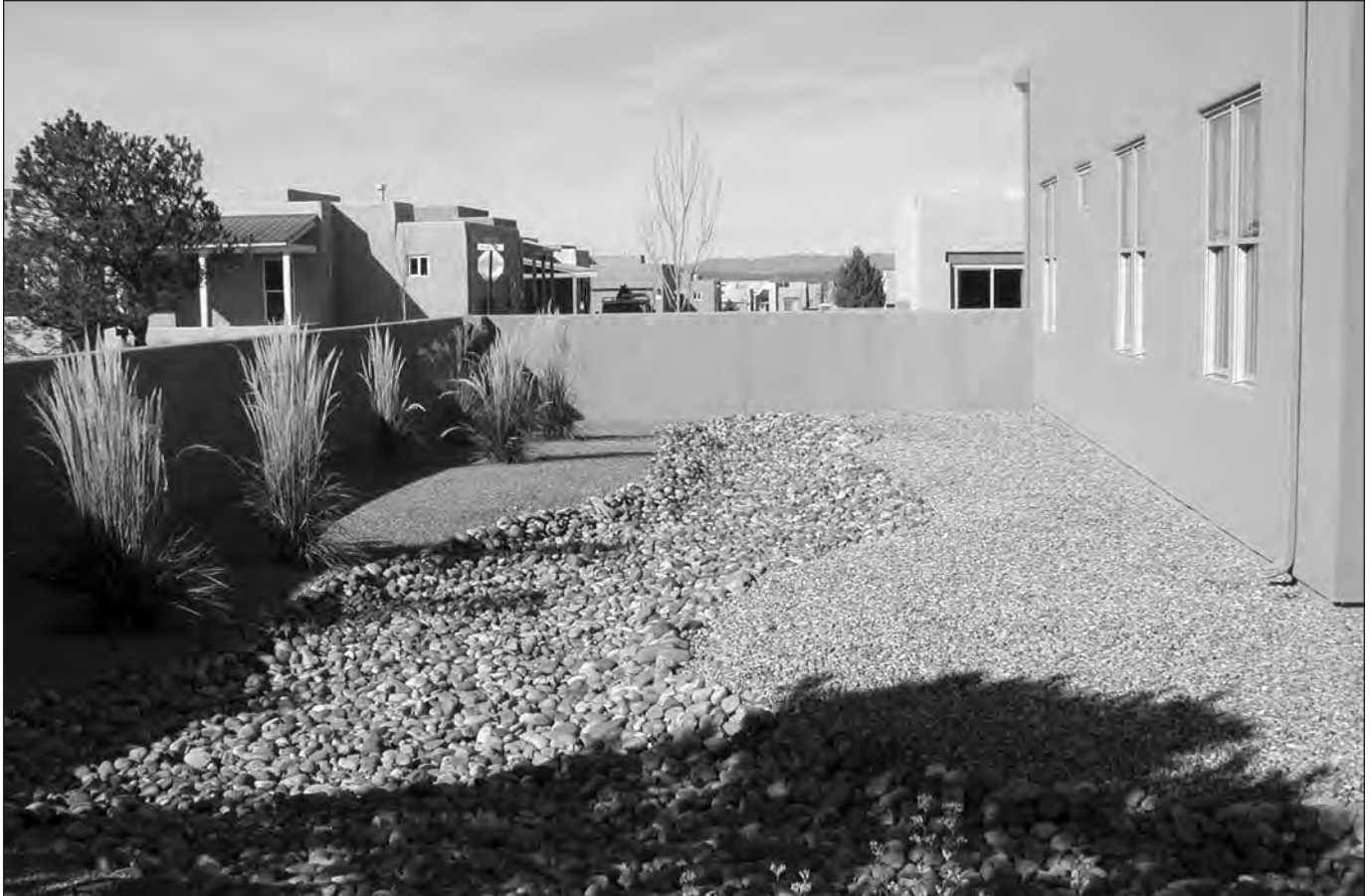
WATER-HARVESTING SYSTEM - COBBLE DRAINAGE WAY AND CRUSHED STONE YARD WINDMILL RIDGE UNIT 1 VISTA SERIES
