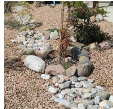
Image 4.15 Stone Erosion Control Techniques
