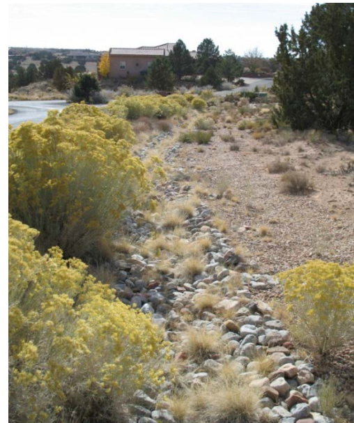
Image 4.35 Open Space Stone Armored Swale
