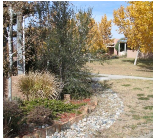
Image 4.5 Rock Swale Passive Surface Water Catchment System
