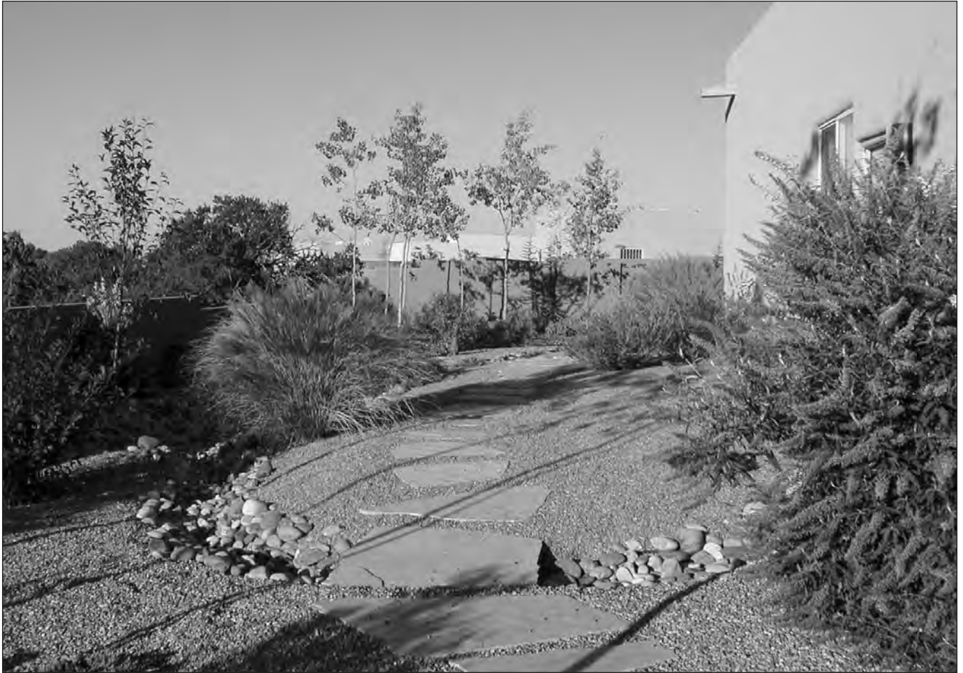
RESIDENTIAL XERISCAPE AND STONE DRAINAGE WAY WATER-HARVESTING SYSTEM THE VILLAGE AT RANCHO VIEJO UNIT I
