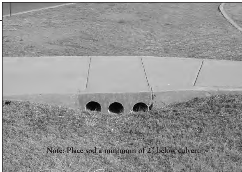
TYPICAL SIDEWALK CULVERT
