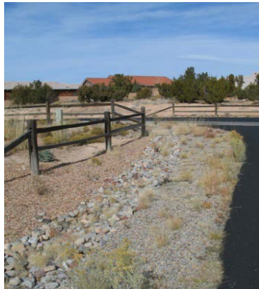
Image 4.33 Roadway Stone Armored Drainage Swales
