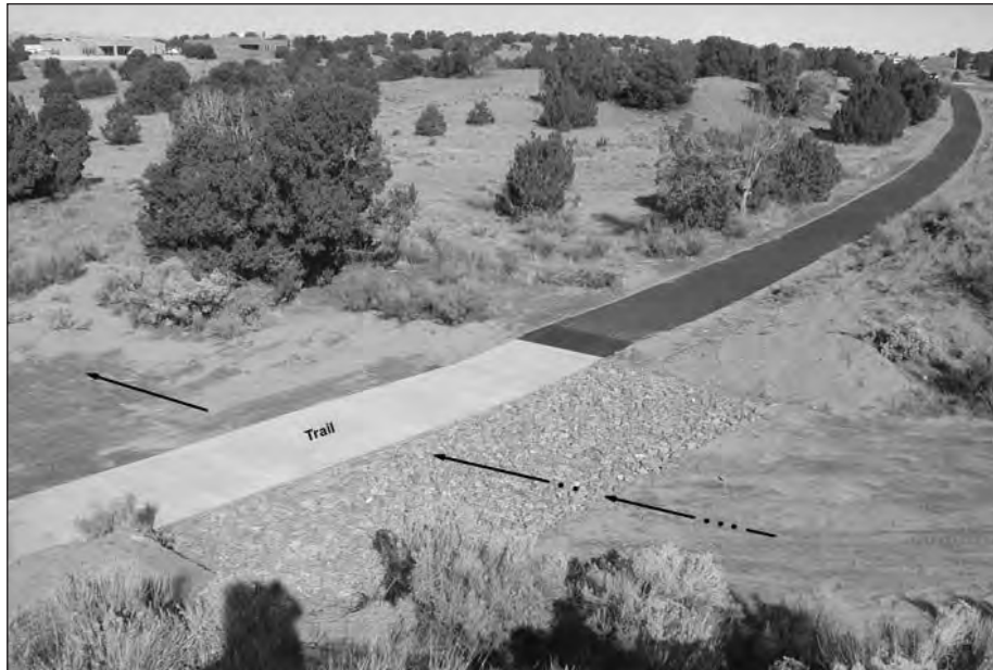
GABION SUPPORTED TRAIL WINDMILL RIDGE - WEST OF RICHARDS AVENUE
