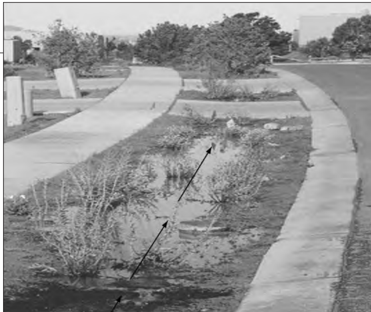
WATER-HARVESTING SWALE IN FLAT-CURBED PARKWAY
