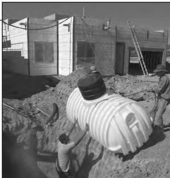
CISTERN INSTALLATION THE VILLAGE AT RANCHO VIEJO
