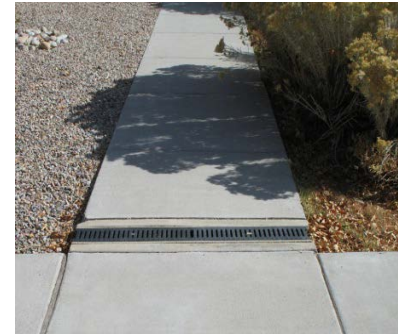
Image 4.14 Paving and Area Drains
