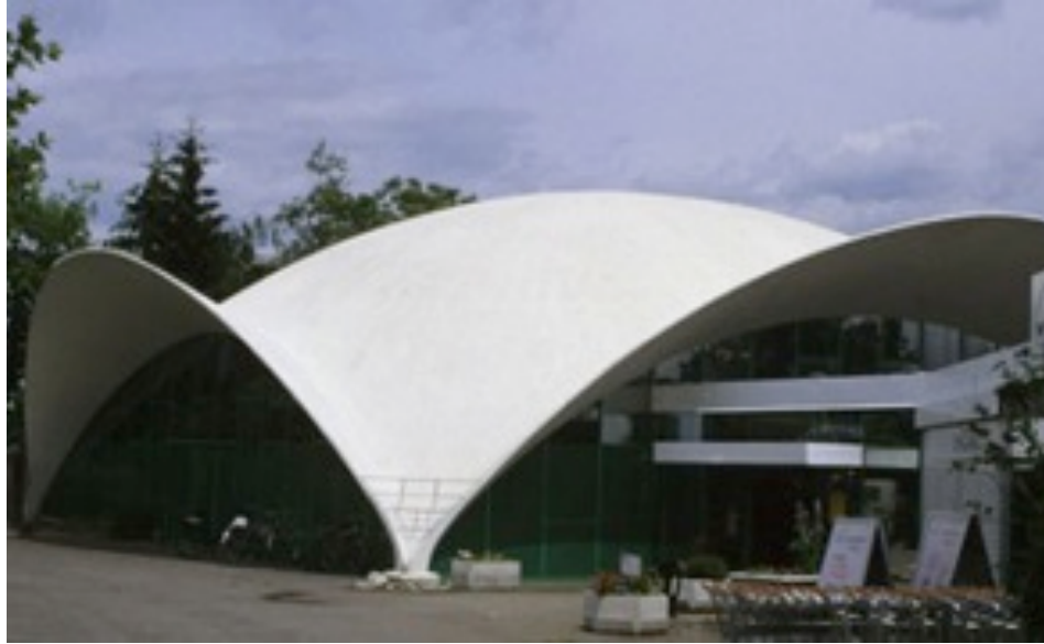
Fig 2.12. Concrete shell by Isler (Chilton, 2000)
