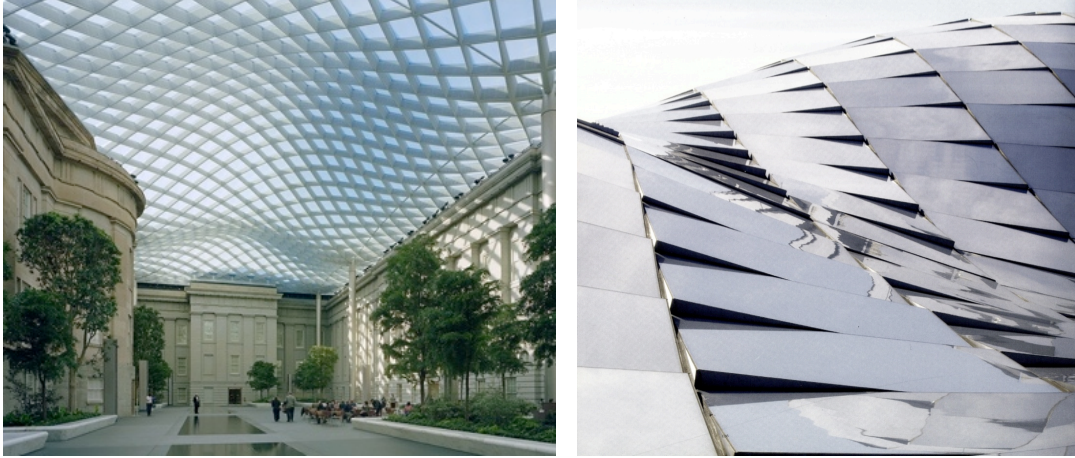
(a) general view of the atrium with the roof top (b) the detail of the gap generated between the panels
