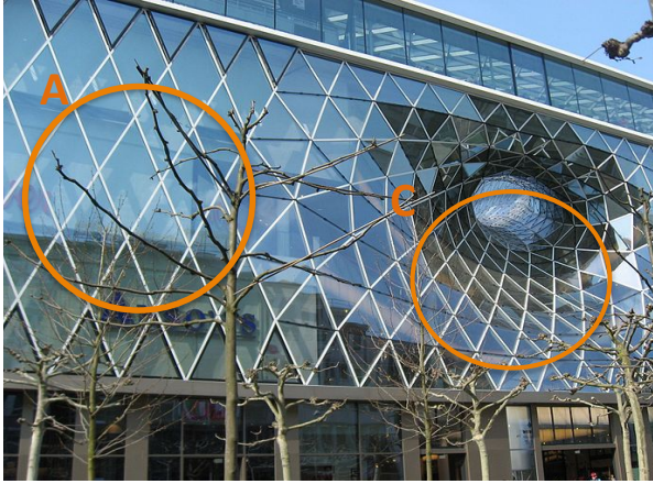
Fig 1.9. MyZeil by Fuksas
