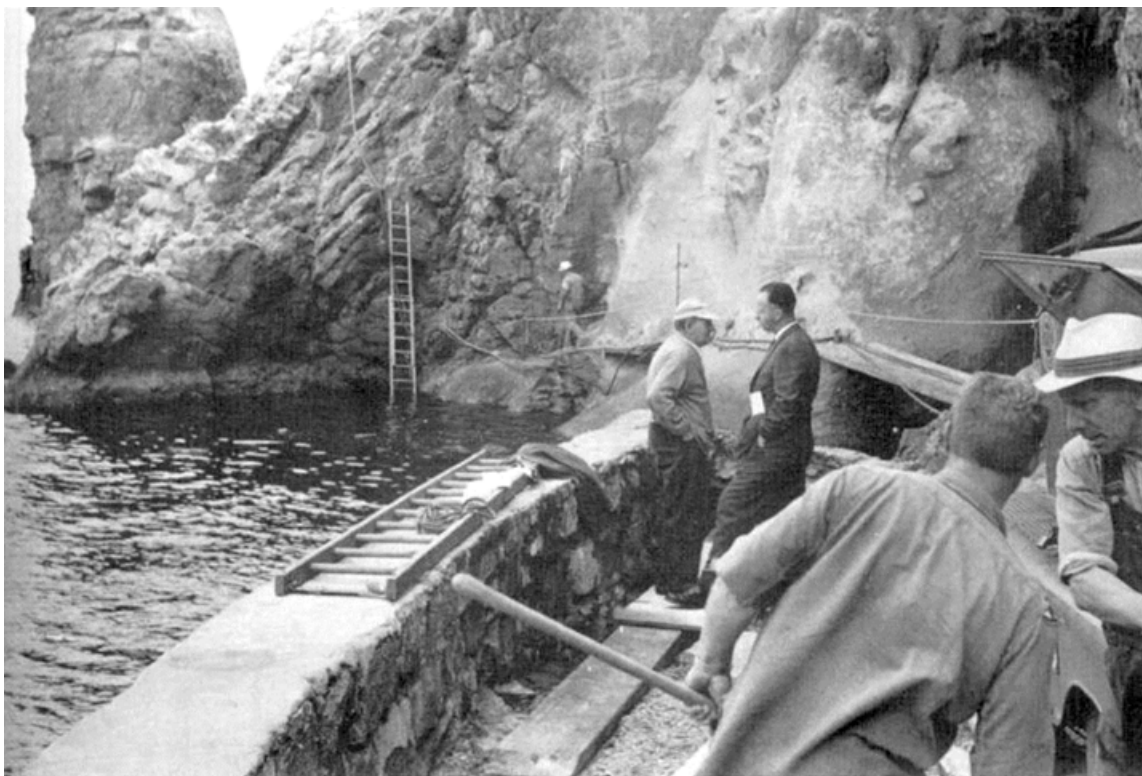
Figure 2.31: Construction on the Seawall, at Siwash Rock, 1963 (Steele, 1993).
