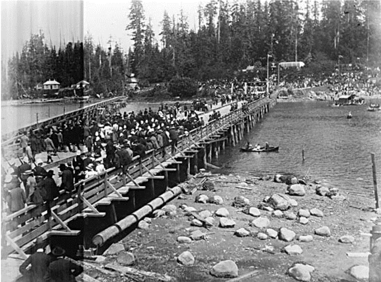
Figure 2.16: Bridge across Coal Harbor to Stanley Park, 1898 (City of Vancouver Archives).
