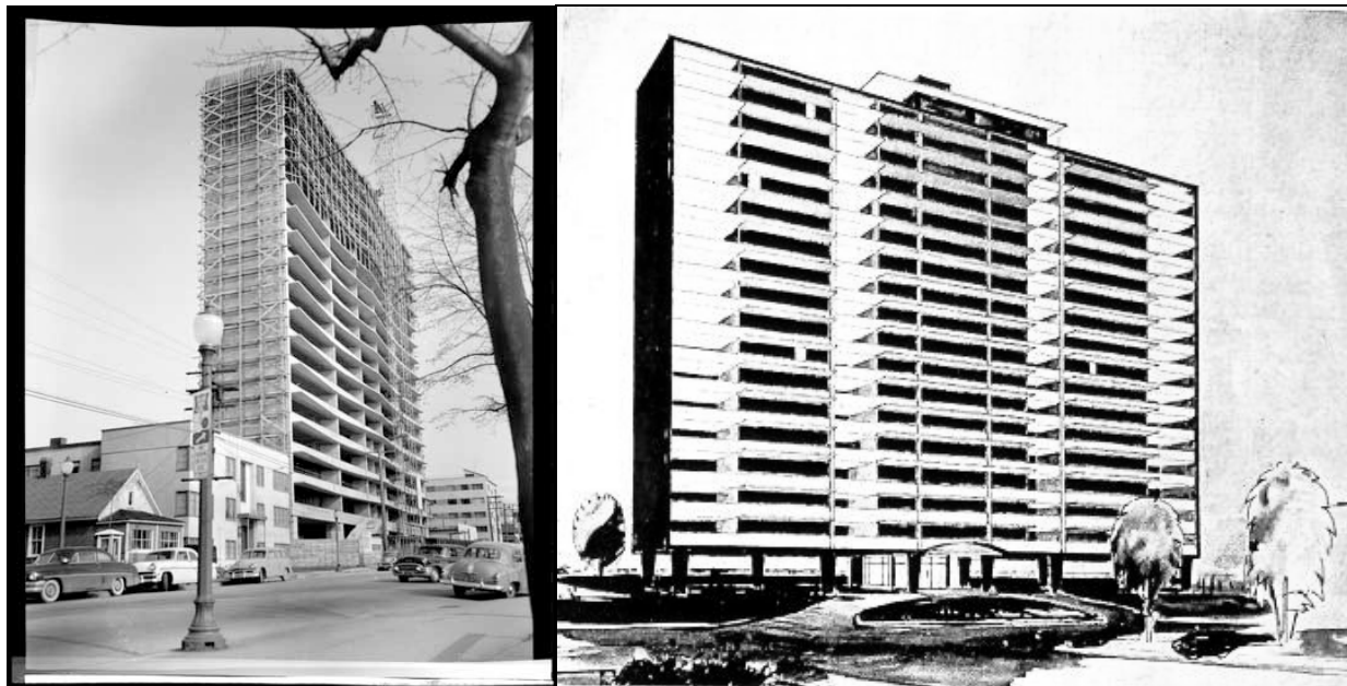
Figure 4.6: Ocean Towers building, shown under construction in 1958 (Vancouver Archives), and as published (Western Homes and Living, June 1958).
