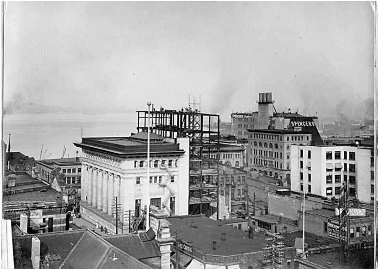
Figure 2.2: Downtown Vancouver in 1910, facing North (City of Vancouver archives). The lower image is an enlargement of the central frame. While the far shore is dimly visible, the view of the towering Coastal Mountains has been hidden.
