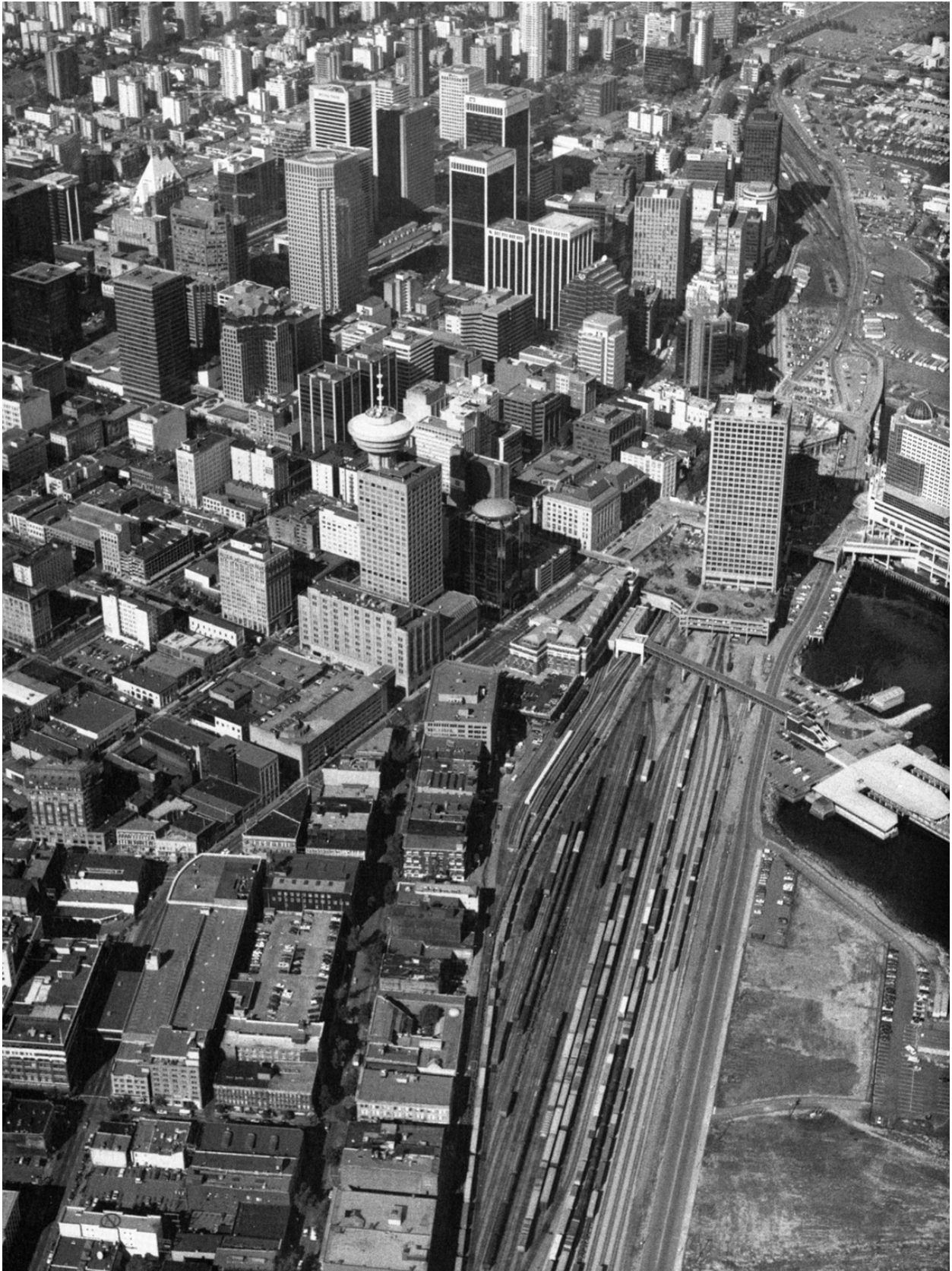
Figure 6.27: An aerial view of the project 200 site in 1992 (Ley, 1992).
