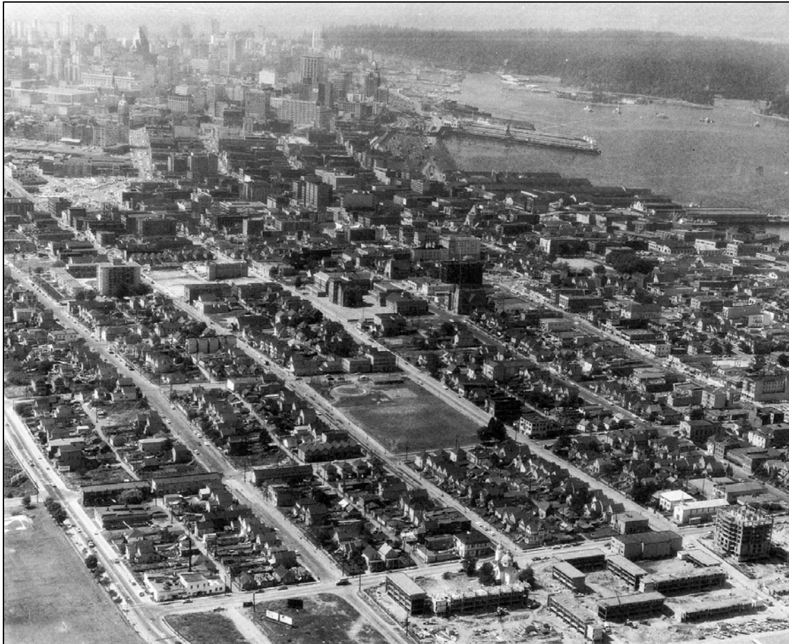
Figure 5.1: Strathcona in 1966, View looking west. (Atkin, 1994) In the distance can be seen the West End and Stanley Park. In the foreground is Raymur Place, under construction.
