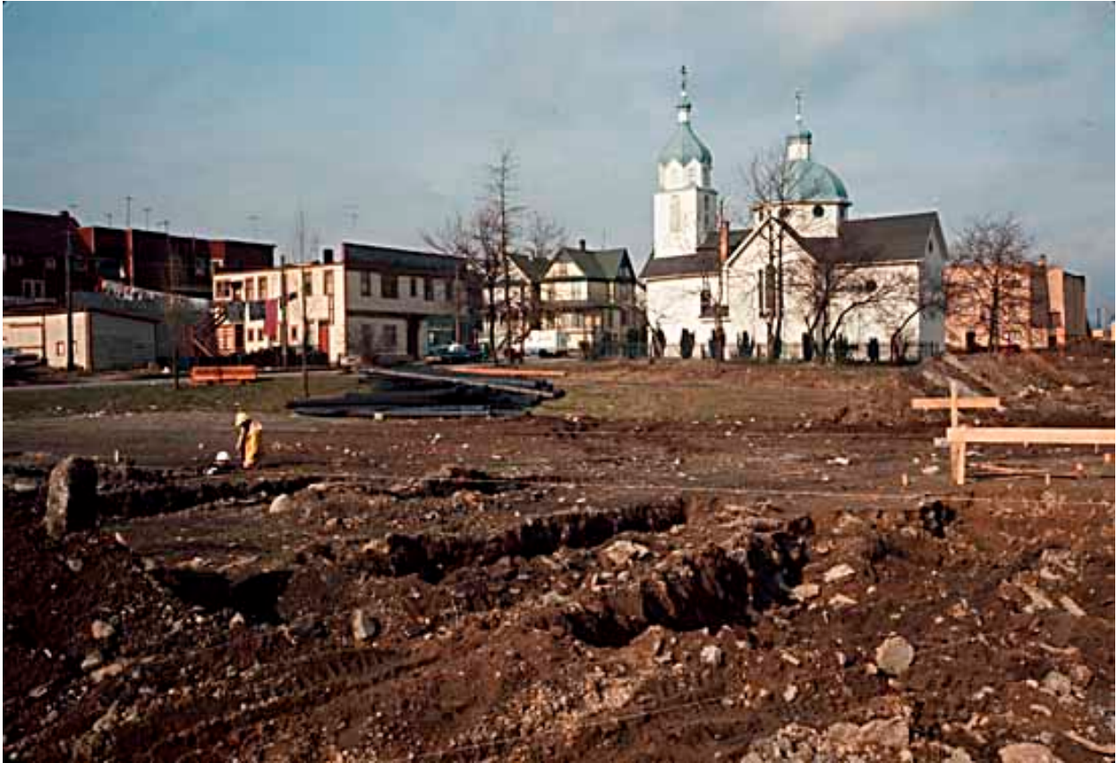
Figure 5.18: Raymur Place: preliminary site work 1966 (City of Vancouver Archives.) Note: for a sense of scale the church preserved in this image and in figure 5.19.
