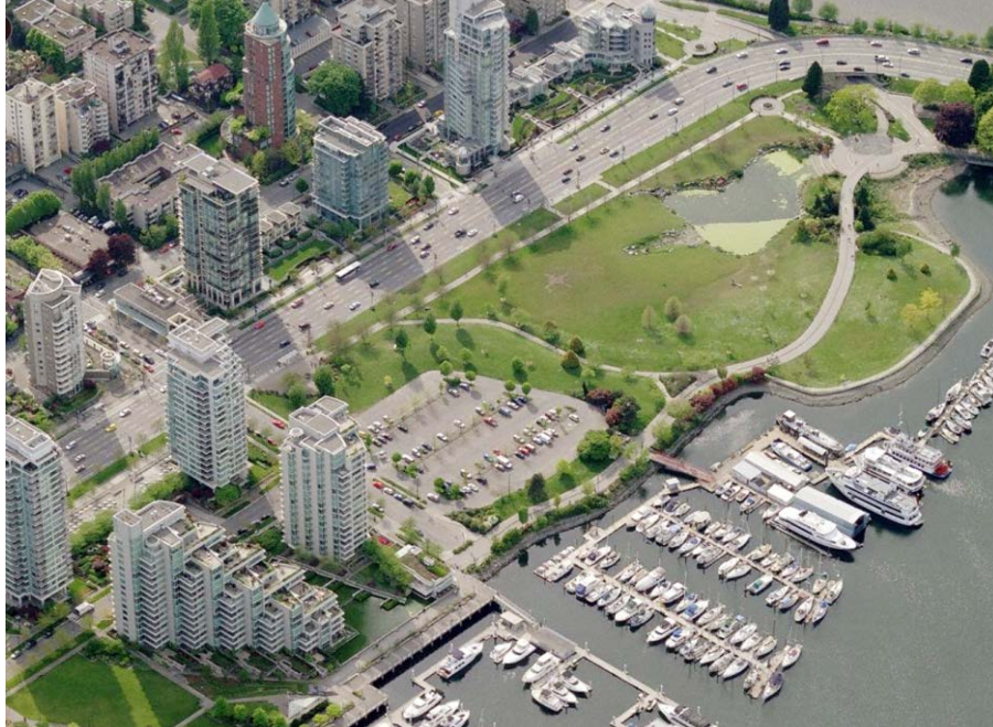
Figure 6.19: Devonian Harbor Park and neighboring developments (Bing 3-d, 2011).
