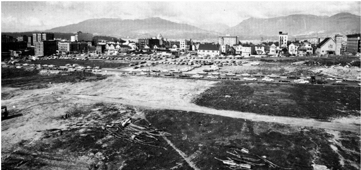
Figure 5.15: Four blocks of homes demolished in Strathcona in 1968 (Marlatt and Itter, 1979, p 178). Although additional information regarding this photograph is scarce, an analysis of existing buildings, and the vantage point of this image suggests that this picture may have been taken standing on the fifth or sixth floor of the tower constructed at Maclean Park in phase I; the work shown here depicts land cleared for phase II. For a view of this area today, see figure 5.16.
